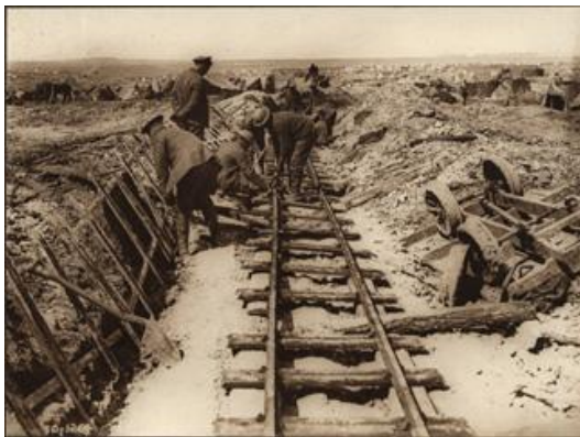
Figure : Canadian Soldiers Building a Light Railway, [ca.1918] 1
