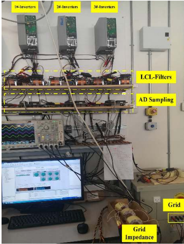
Fig. 19. Hardware picture of the experimental setup with three paralleled inverters.
