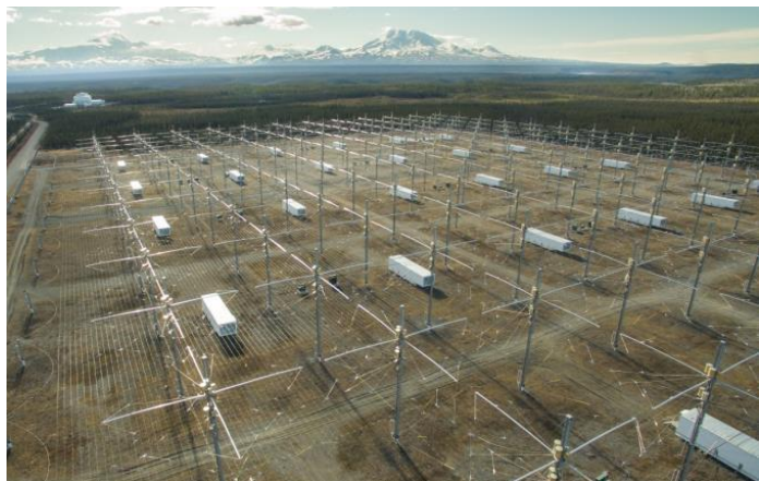
Figure 2.1. HAARP antenna array. Drone photo courtesy of Jessica Matthews.
