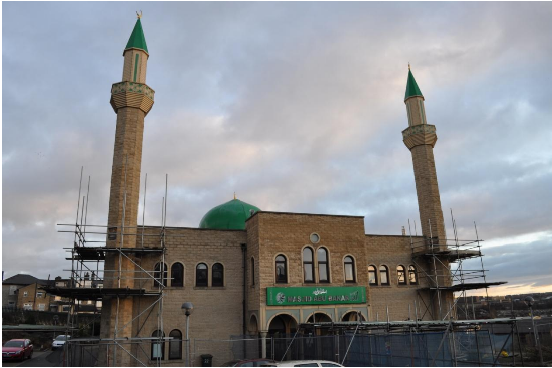
Picture 3-1: Surveys were conducted at the Abu Bakr Mosque on Steadman Terrace Road (Reid, 2010)
