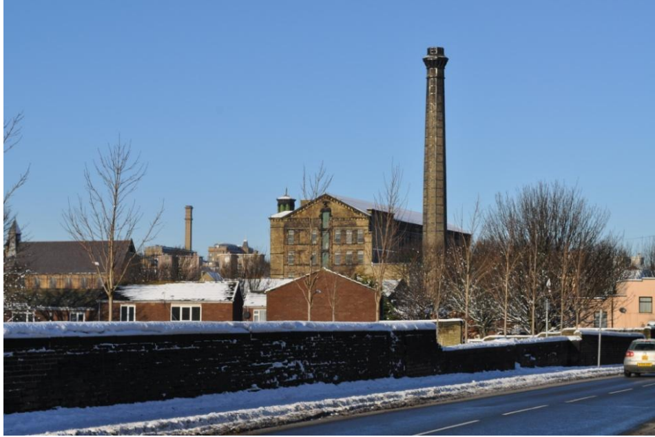
Picture 3-7:Victorian-era woolen mills still dot Bradford's cityscape. Drummonds Mill in the foreground, Lister Mill in the background (Reid 2010)
