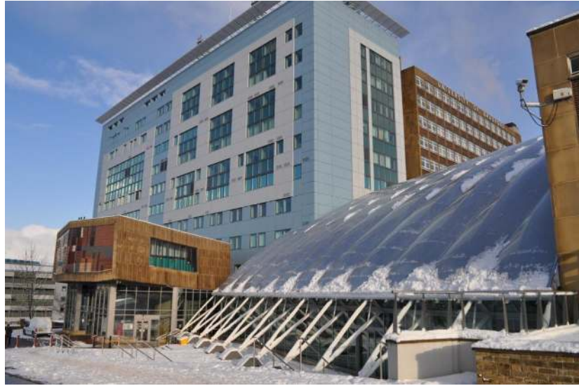
Picture 3-10: Atrium and Richmond Building, University of Bradford (Reid, 2010)
