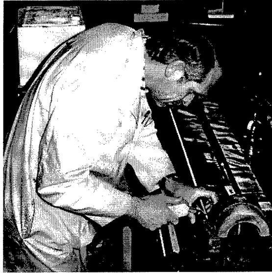
Figure 3 : Wick Fabrication
