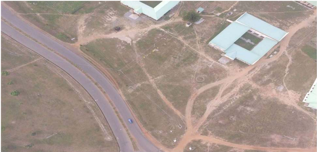
Figure 4a: UAV acquired image of part of FUTMinna, Main Campus (reference image)
