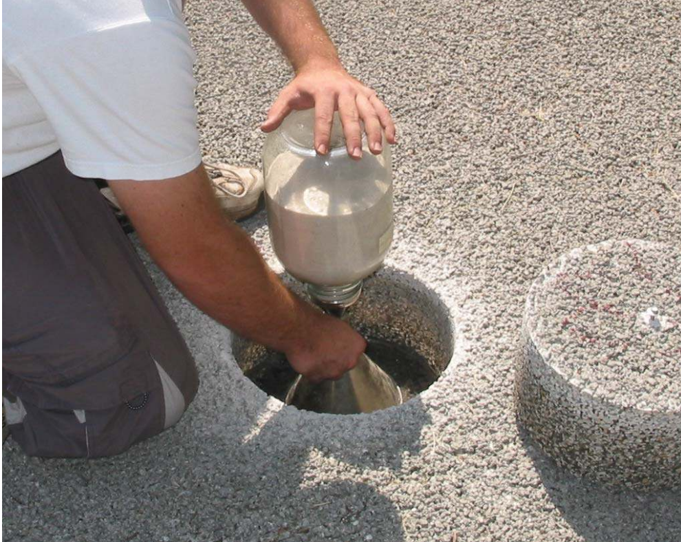
Figure 10: Performing Sand Cone Test
