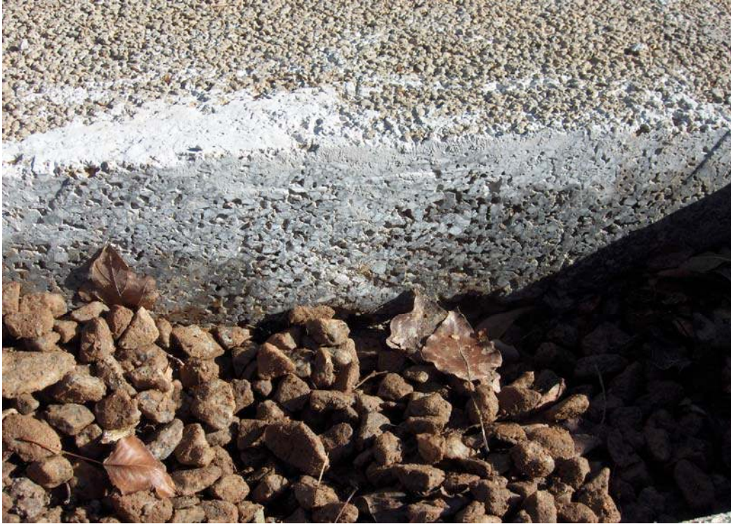
Figure 32: Cleveland Park Parking Lot Reservoir
