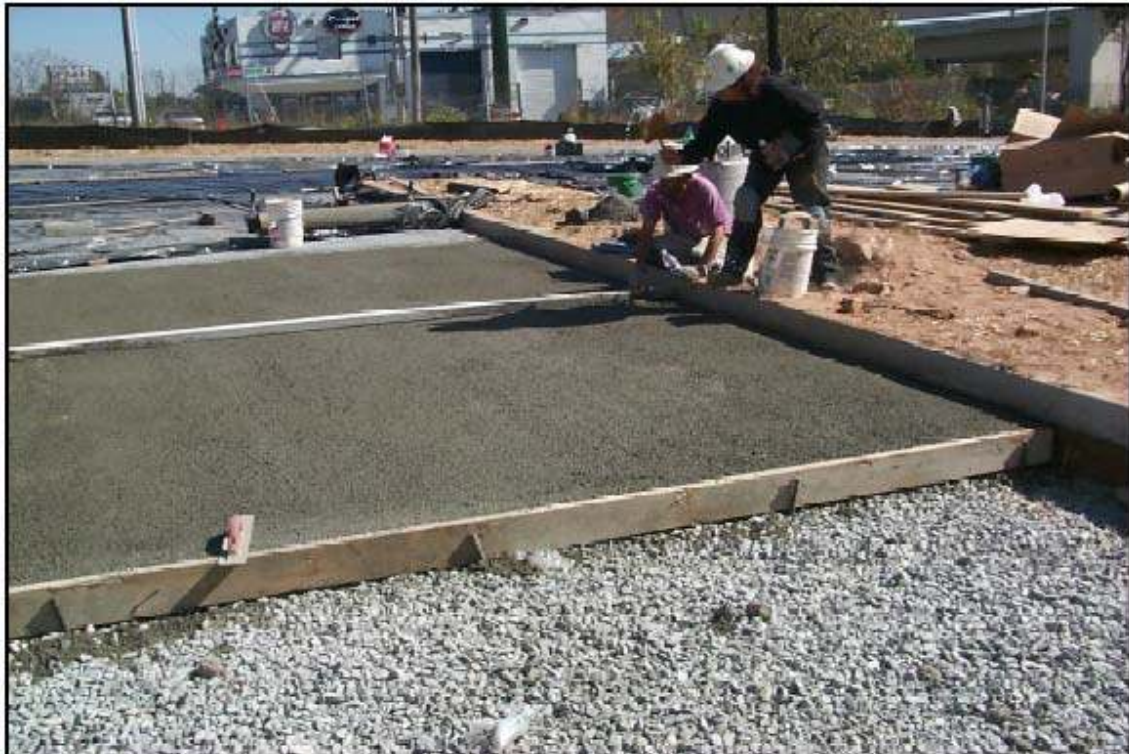
Figure 2: Typical Porous Concrete Installation
