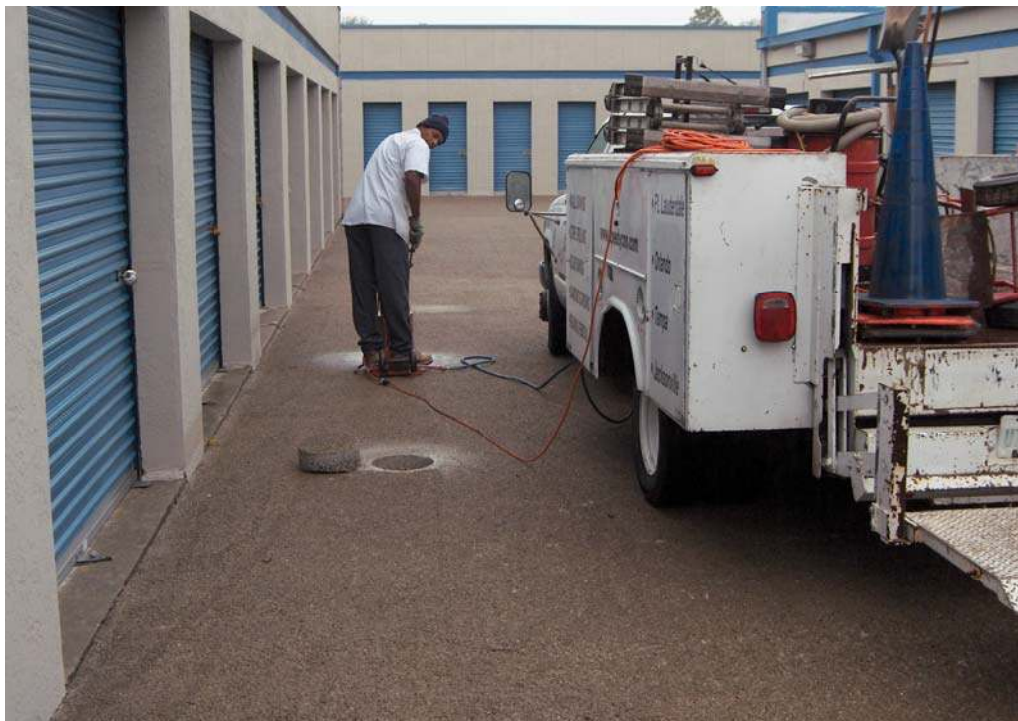
Figure 16: Sun Ray Store-Away Pervious Pavement at Core Locations 1, 2 & 3
