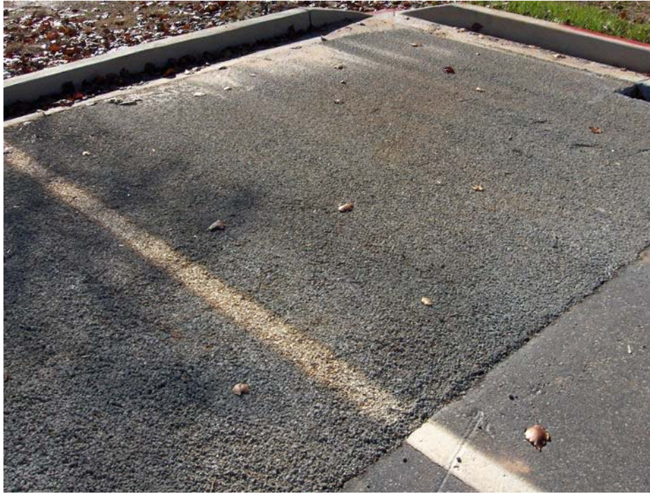
Figure 31: Cleveland Park Parking Lot Pavement
