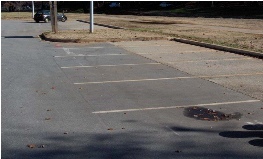
Figure 30: Cleveland Park Parking Lot
