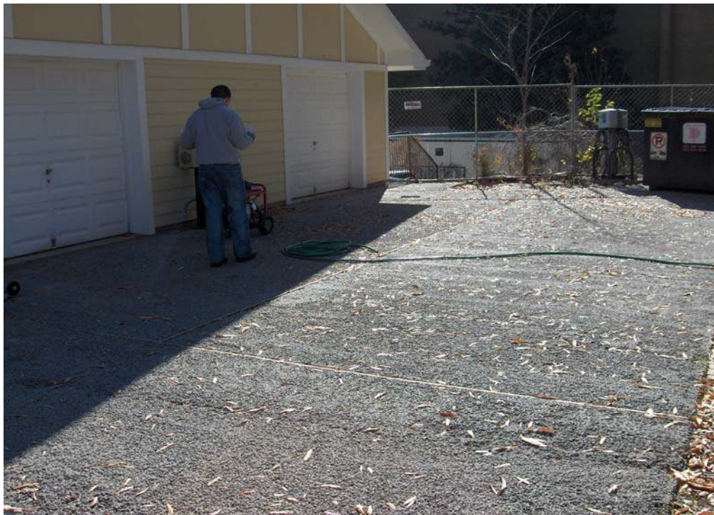
Figure 28: Southface Institute Parking Lot
