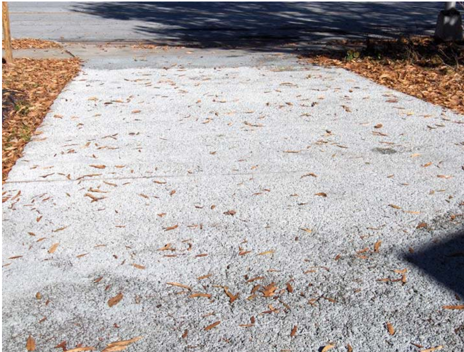
Figure 26: Southface Institute Parking Lot
