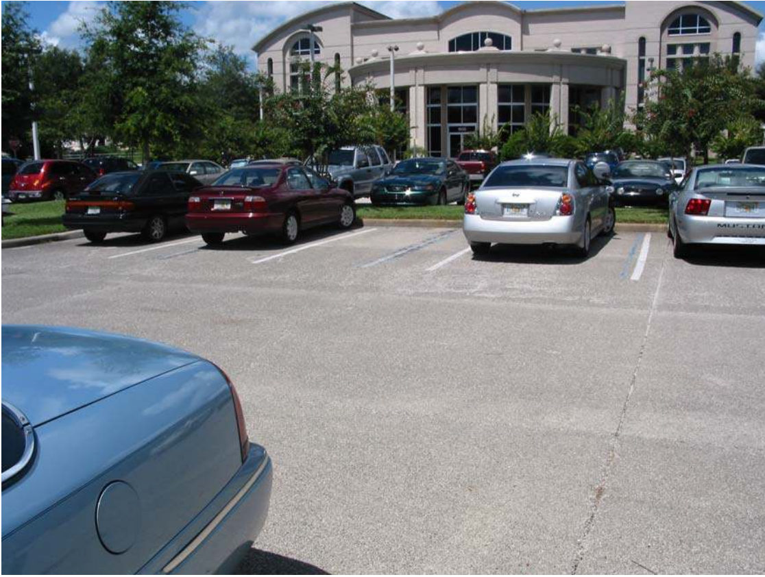
Figure 18: Strang Communication Office Parking Lot
