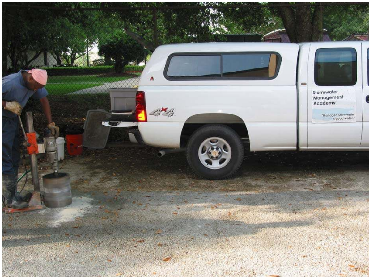
Figure 22: FDEP Parking Lot Core Test
