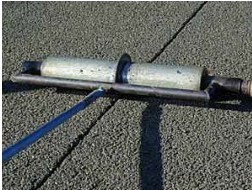
Figure 43: Roller Used to Create Joints in Pervious Concrete
