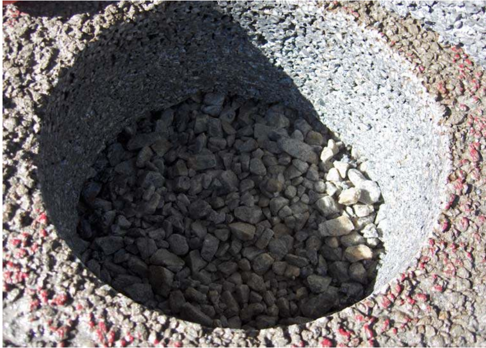
Figure 27: Southface Institute Gravel Subbase
