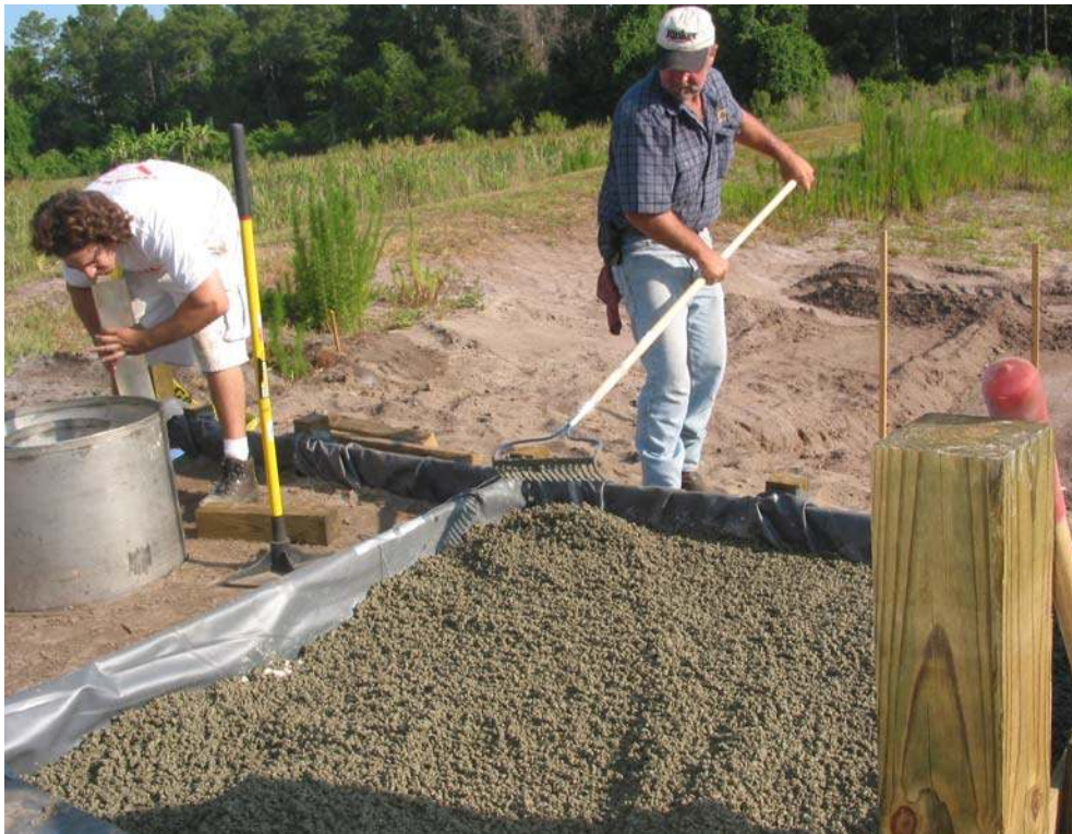
Figure 3: Stormwater Academy Porous Concrete Test Cell Installation
