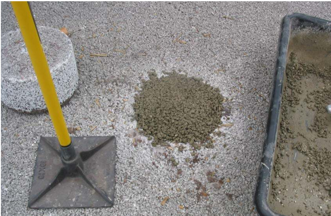
Figure 11: Repair of Concrete Core Area
