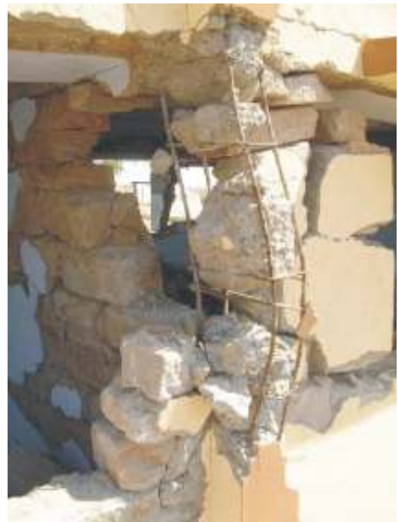
Fig. 25. Details of the short columns in the building shown in Fig. 24.
