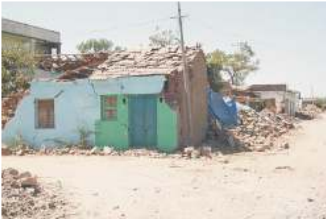
Fig. 5. A village house in Kachchh; stone masonry with Manglore tile roof.
