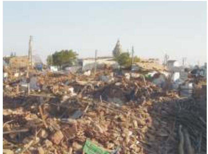
Fig. 7. Virtually complete destruction of masonry buildings in a village in Kachchh.
