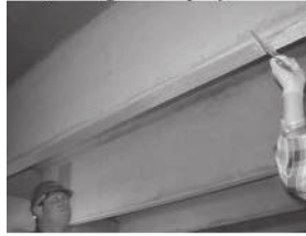
c) Squeezing Out the Resin Excess
