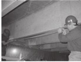
d) Application of Scrim on Longitudinal Ply
