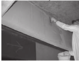
f) Application of Epoxy on U-Wrap
