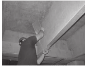
e) Application of U-Wraps
