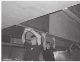
b) Application of Longitudinal Ply
