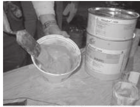
a) Mixing of the Epoxy Resin
