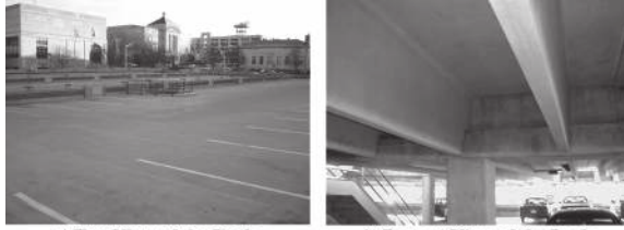
a) Top View of the Deck
