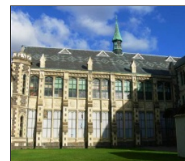
(c) Engineering building
