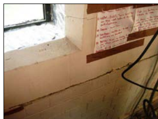
a) Out-of-plane rocking resulting in residual displacement along North elevation of 10 mm
