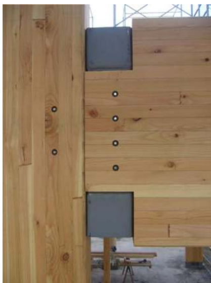
Fig. 2 LSB connections
