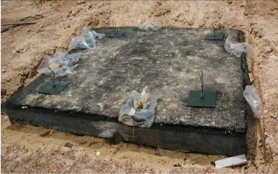
Figure 17. Completed SHS multi-layer pavement slab with anchoring at site
