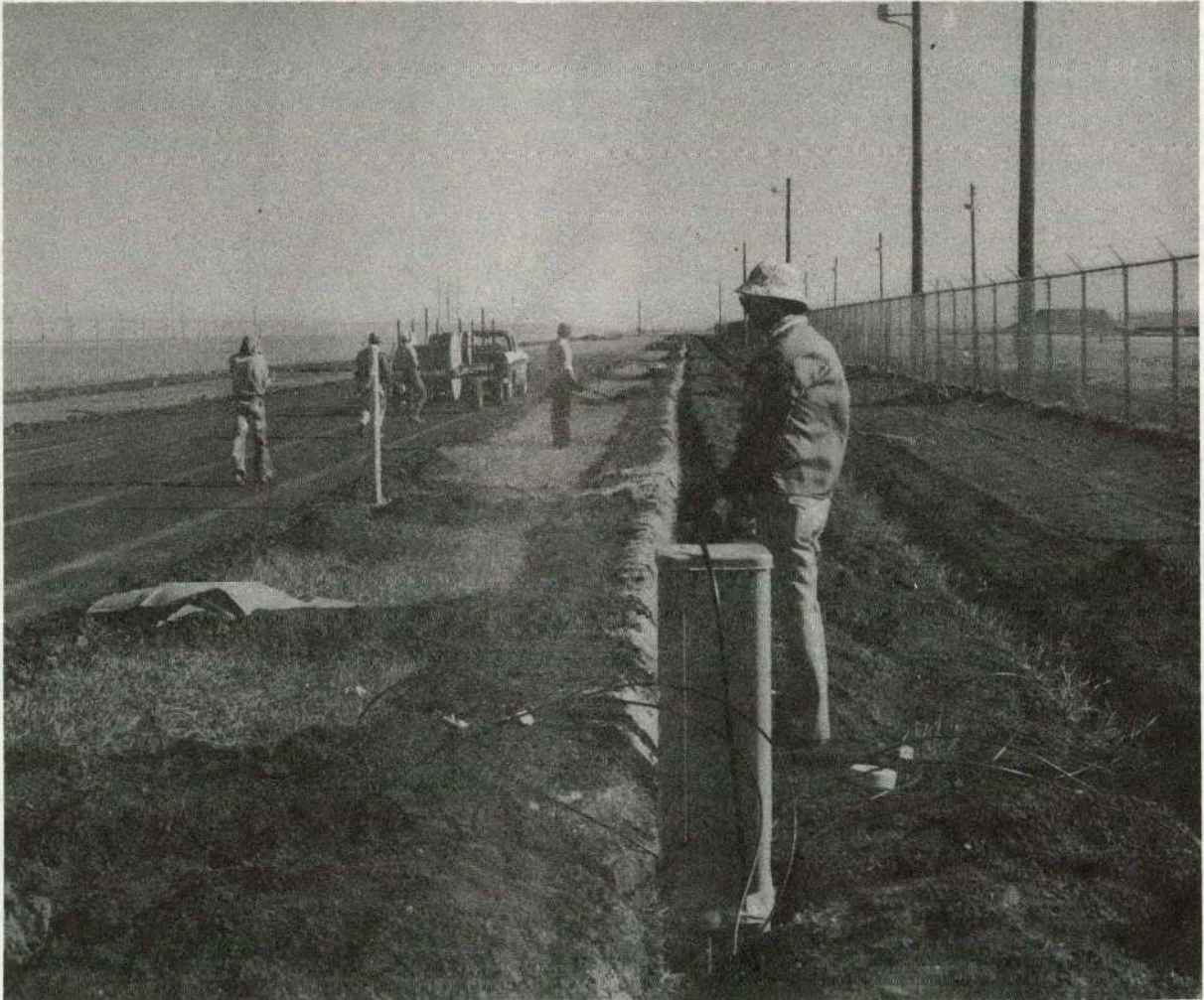
Figure A-2. Site Construction Activity
