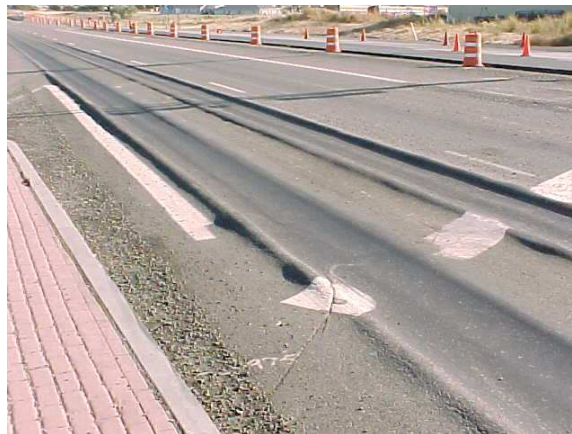
Figure 1.1 Definition of permanent deformation (source WAPA)
