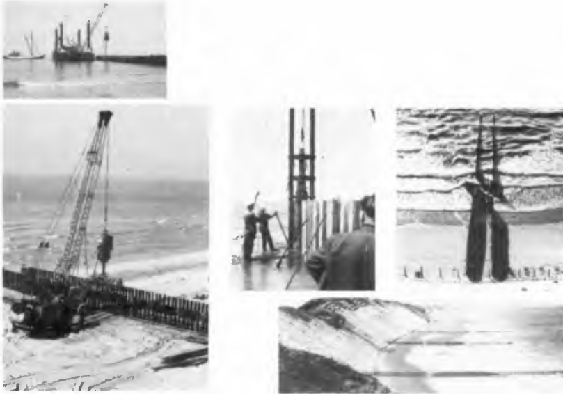
FIG.8 Construction of screens
