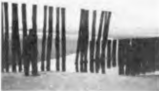
FIG.18 Pulled piles
