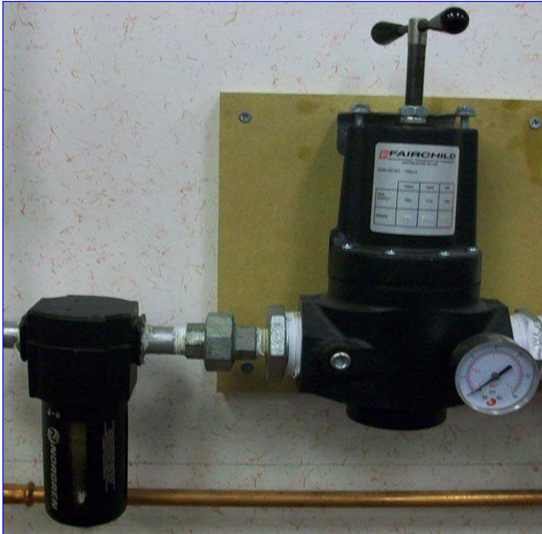
Figure 5.6 FAIRCHILD Flow Pressure Regulator
