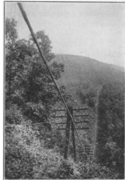
FIG. 10—CABLE LINE ON STEEP SLOPES
