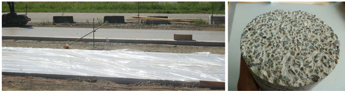
Fig. 11 Trial section of double layered concrete with \text{TiO}_2 in the top layer on industrial zone “Den Hoek 3” in Wijnegem
