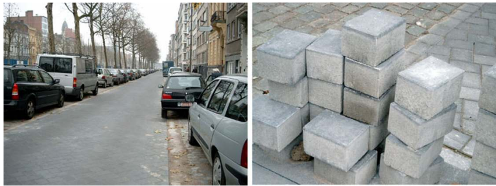
Fig. 5 Separate parking lanes at the Leien of Antwerp with photocatalytic pavement blocks
