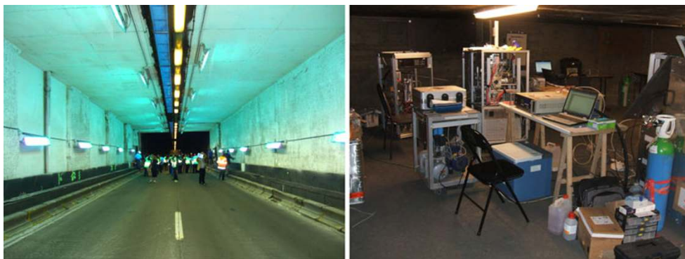
Fig. 10 Leopold II tunnel test site, after renovation in September 2011 and dedicated testing equipment
