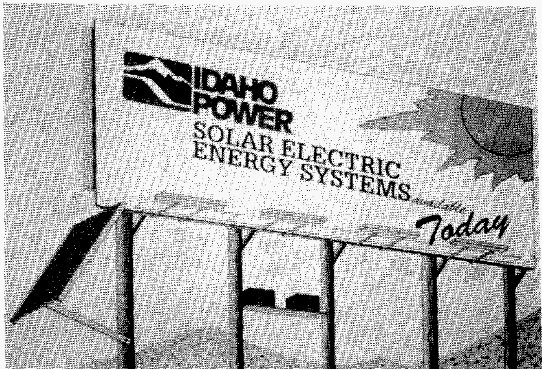
Figure 3. Idaho Power PV Installation
