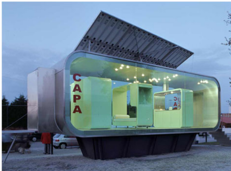
Figure 10. CAPA, Matosinhos, Portugal, 2003. The PV generator is shaped as a sloped plane that characterizes the image of the building. Design: Cannatà & Fernandes. Picture ©Cannatà & Fernandes
