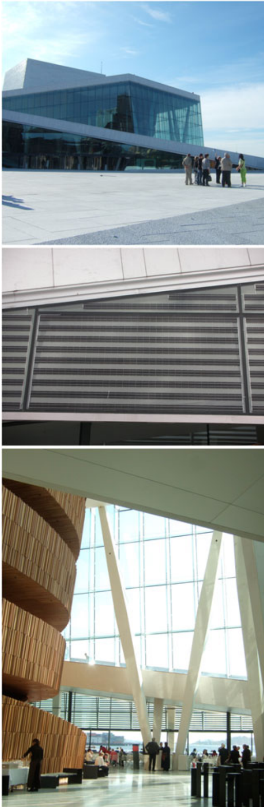
Figure 6. Opera House, Oslo, Norway, 2008. The long triangular band above people's head is the glass part where the 400 m 2 solar PV is mounted in a pattern made of cells strips. Design: Snøhetta. Pictures ©H. N. Røstvik and A. Scognamiglio.
