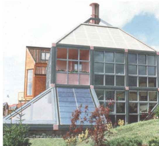
Figure 8. Chanelle House, Stavanger, Norway, 1988. PV is used together other solar technologies, and its influence on the building's image is quite limited. Design: H. N. Røstvik. Picture ©H. N. Røstvik.
