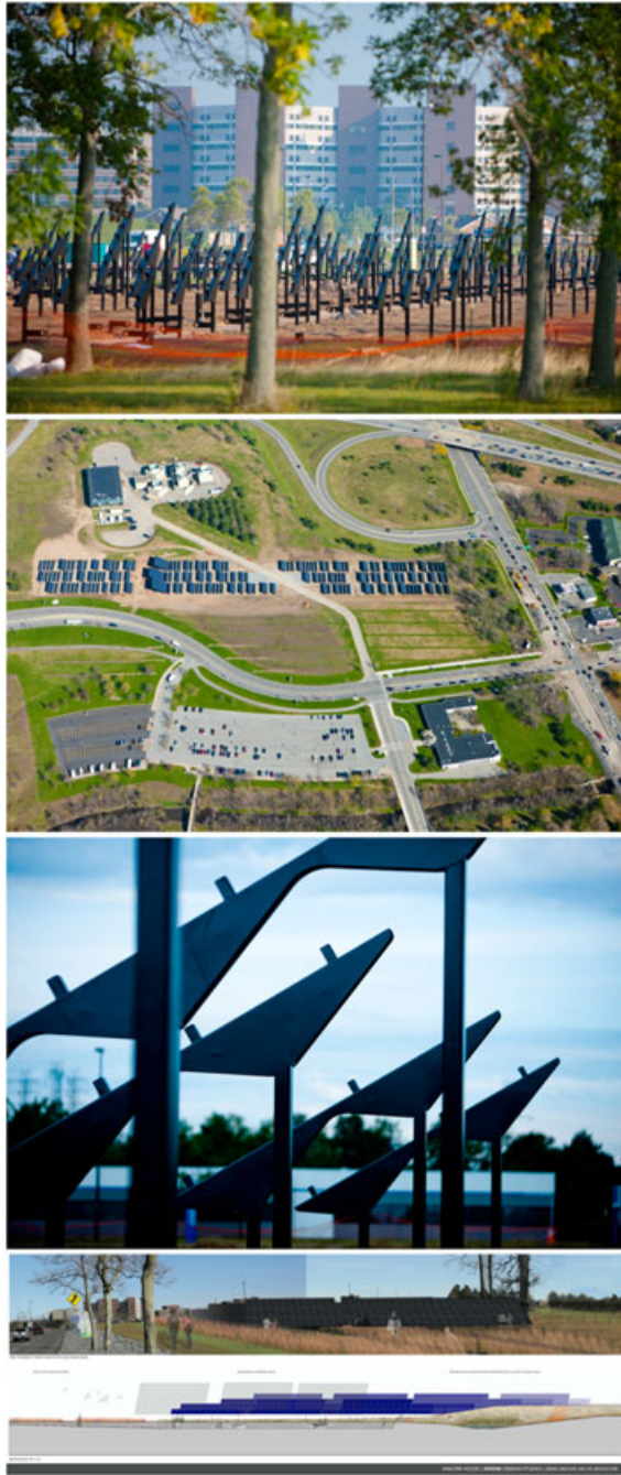
Figure 18. The Solar Strand, Buffalo University Campus, Buffalo (US), 2011. The PV modules on the ground are arranged according to a DNA pattern. They give form to a public space in a direct functional and visual relationship with the buildings of the campus. Design: Walter Hood, Hood Design. Pictures by courtesy of the architect ©W. Hood.
