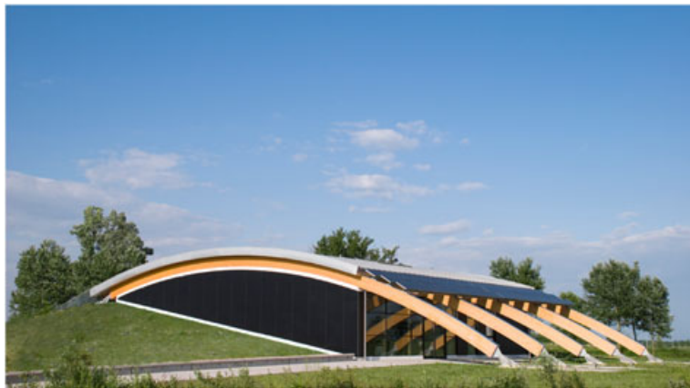
Figure 4. Polins, Portogruaro (new building), Italy, 2010. PV is part and parcel of the curved sun-shading system of the southern facade. Design: Marco Acerbis. Picture by courtesy of the architect ©M. Acerbis.
