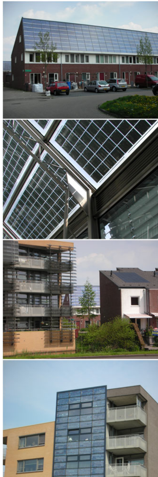
Figure 1. Examples of different ways of integrating PV in (or adding PV to) the building envelope (rooftops, semitransparent envelopes, sun-shading and cladding). Pictures ©A. Scognamiglio.
