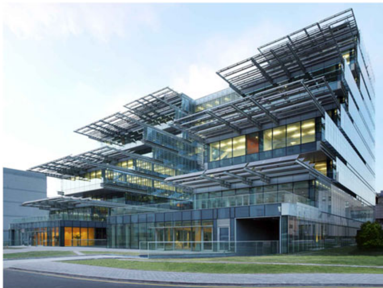
Figure 14. SIEEB building, Beijing, China, 2006. PV modules are arranged as wings that perform as sun-shading devices and give form to a kind of semitransparent half-pyramid. Design: MCA Mario Cucinella Architects. Picture ©MCA Architects.
