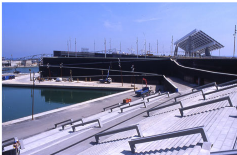
Figure 2. Forum 2004 Esplanade and Pergola, Barcelona, Spain, 2004. PV helps in defining the landmark function of the Pergola. Design Torres & Lapeña. Picture by courtesy of the architects ©Torres & Lapeña.
