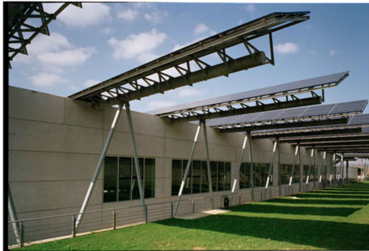
Figure 13. Rainbow Headquarters, Loreto, Italy, 2011, PV modules are arranged as wings hanging over from the building's boundary. Design: S. Bianchi & E. Straffi. Picture by courtesy of the architects ©L. Filateci.
