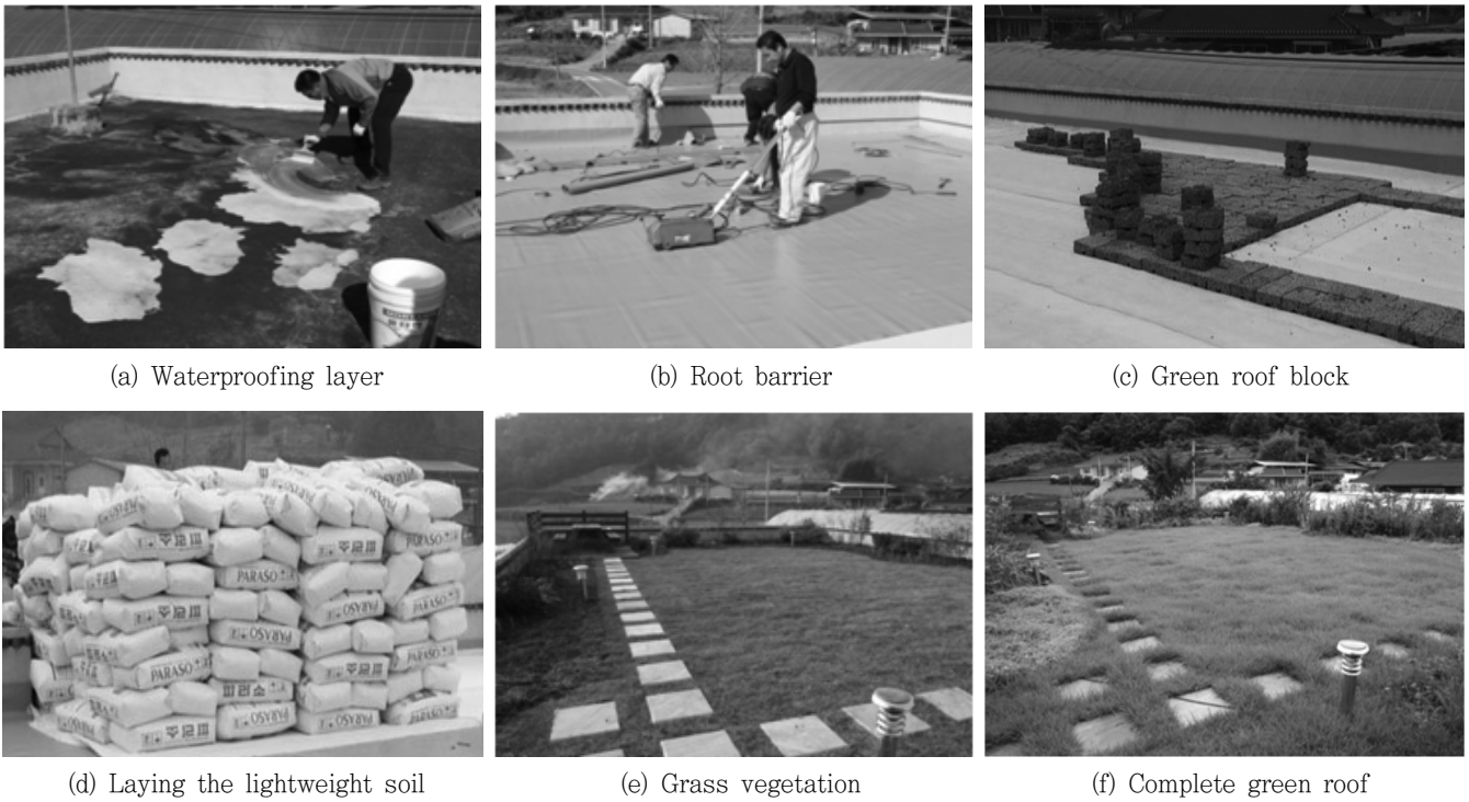
Fig. 2 Process of green roof construction
