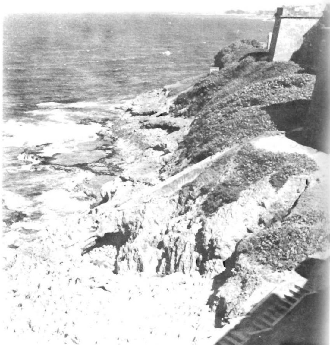
Figure 6. Typical eroded condition of slopes surrounding El Morro castle.
