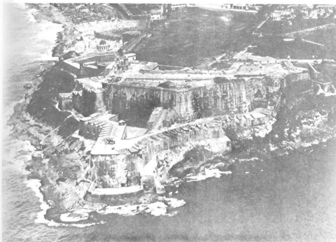
Figure 5. Aerial photograph of El Morro Castle.
