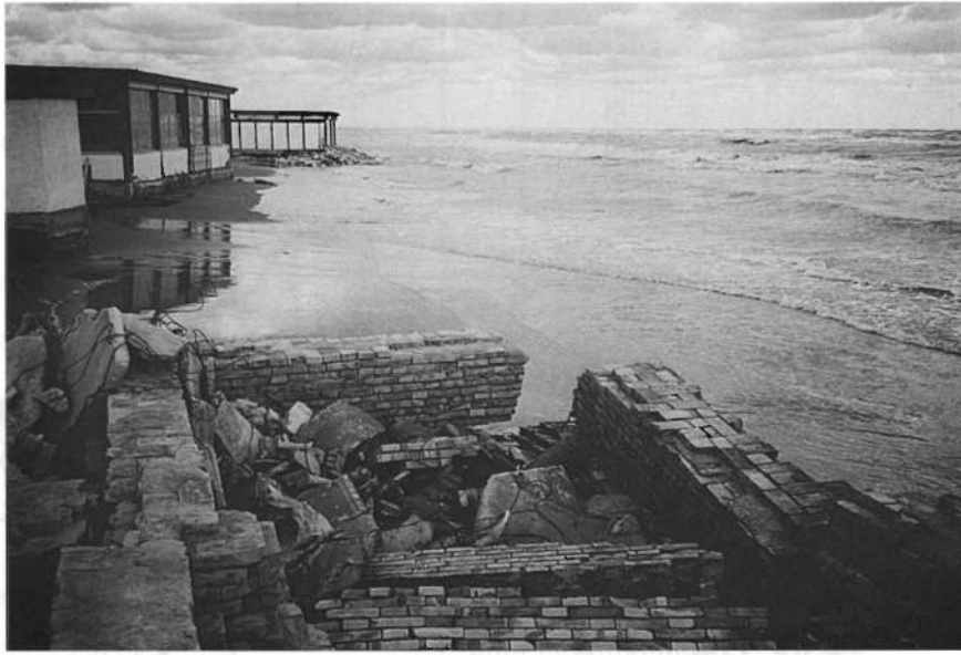
Figure 15. Beach establishment ( bagni ) damaged by erosion at Lido di Dante, south of the Po delta, in the 1980s.
