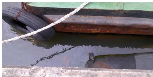
Fig. 1. LNG drainage system (waste discharge point) (point A)
