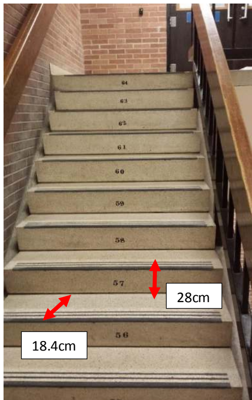
Figure 4: Typical numbered staircase that the SC SIT sessions were performed on. The participant ran up the stairs as fast and as safe as possible using the handrail if necessary for a total of 15 secs, which represented the completion of one work interval. The average step height and step width were 18.4cm and 28cm respectively as indicated by the arrows. Each step was numbered to give an indication to the participant and investigator the step reached upon completion of each 15-sec interval.
