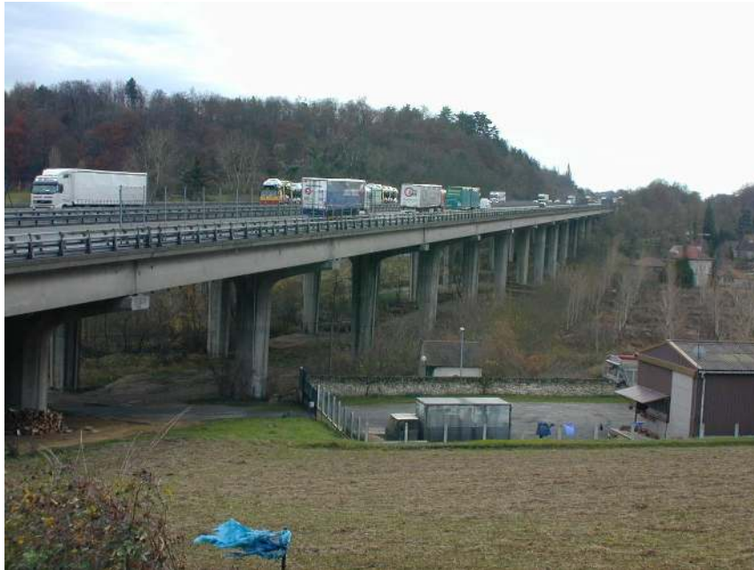
Figure 1. Bridge considered in the study.
