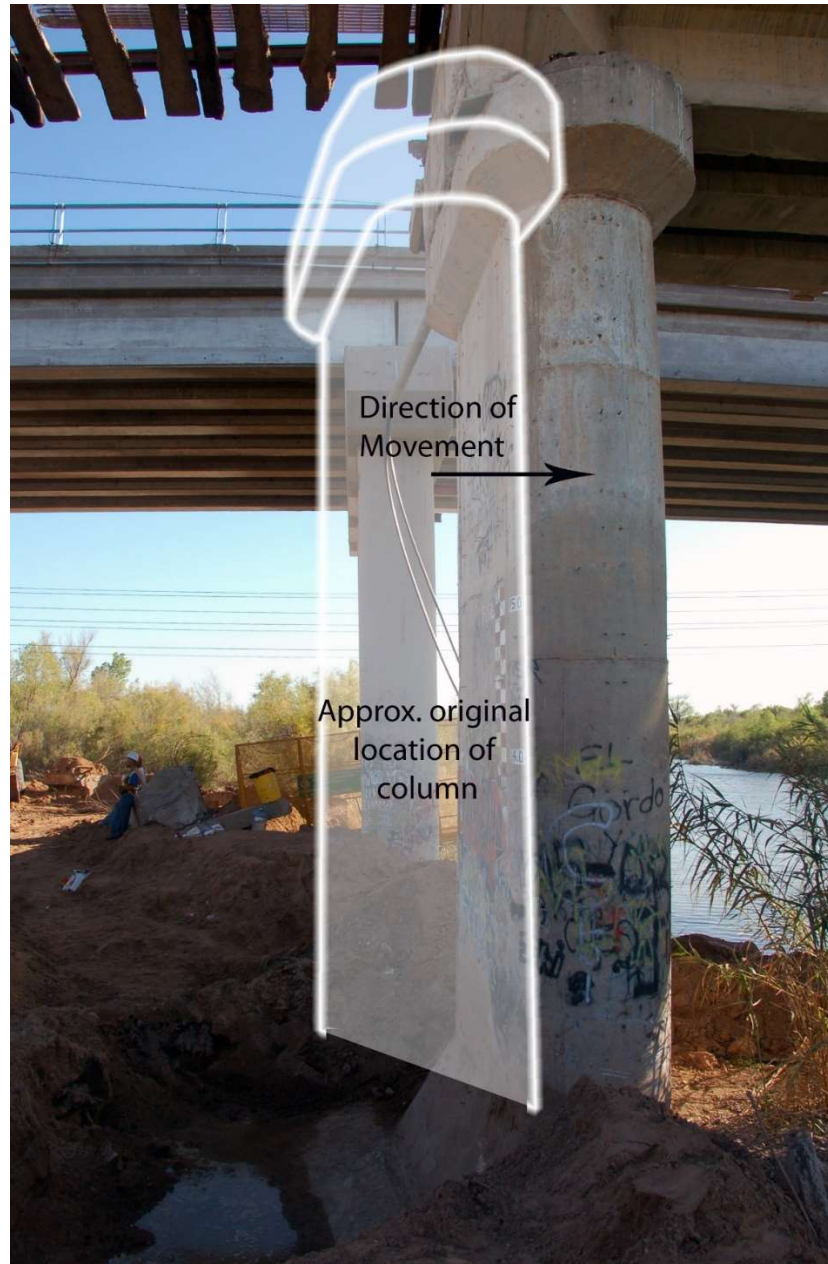
Figure 3: Bent 5 of railroad bridge (foreground) that translated towards river causing unseating collapse, and Bent 5 of highway bridge (background) following 2010 El Mayor-Cucapah earthquake. Photo J. Gingery/GEER (2010).
