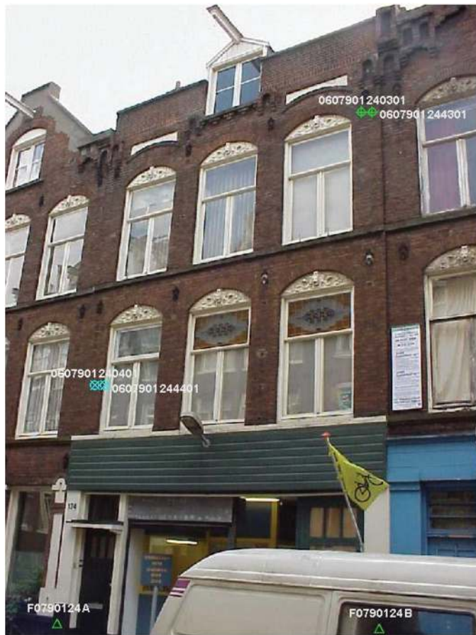
Fig. 16. (Color) Façade with monitoring points for Govert Flinckstraat 124 (Ceintuurbaan) (reproduced by permission of Frank Kaalberg, Witteveen+Bos)
