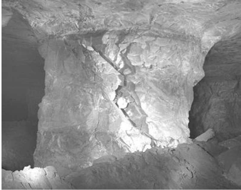
Figure 4. Partially benched pillar that failed along two angular discontinuities. Width-to-height ratio is 0.58 based on full benching height; average pillar stress is about 4% of the UCS.
