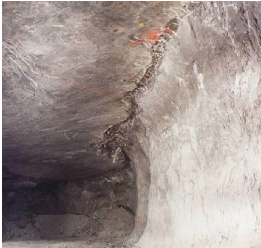
Figure 31. Roof guttering at the pillar-roof contact.
