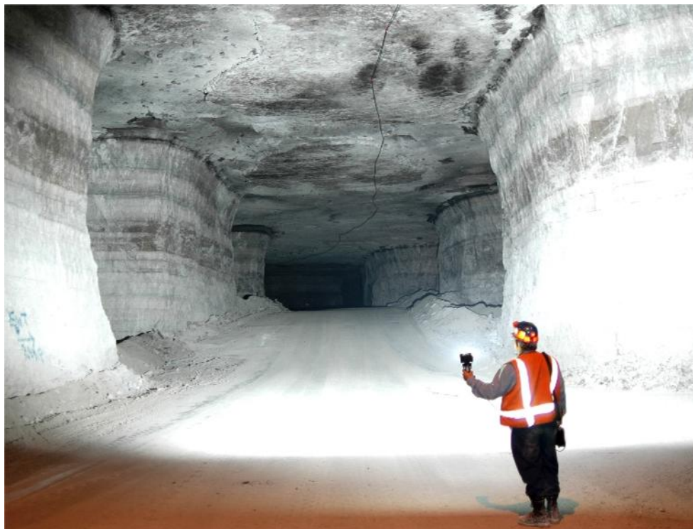
Figure 8. Stable pillars in a limestone mine at a depth of cover of 275 m (900 ft). Slightly concave pillar ribs formed as a result of minor spalling of the hard, brittle rock.
