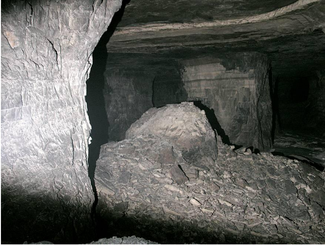
Figure 6. Remaining stump of a collapsed pillar in an abandoned area. Thin, weak beds in the pillar and moist conditions are thought to have contributed to the failure. The width-to-height ratio was 0.82 and average pillar stress about 11% of the UCS.
