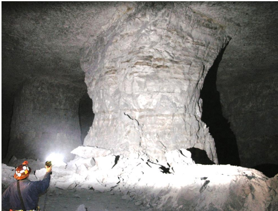
Figure 3. Partially benched pillar failing under elevated stresses at the edge of bench mining. Typical hourglass formation indicates overloaded pillar. The width-to-height ratio is 0.44 based on full benching height and the average pillar stress is about 12% of the UCS.
