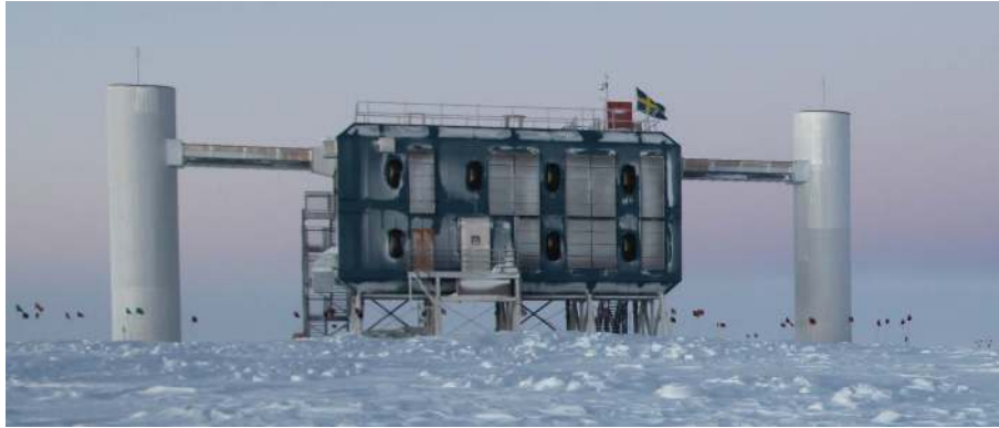
Figure 1: The IceCube Laboratory building houses power, communications and data acquisition systems for IceCube and other experiments at the South Pole (photo by S. Lidström, IceCube/NSF).
