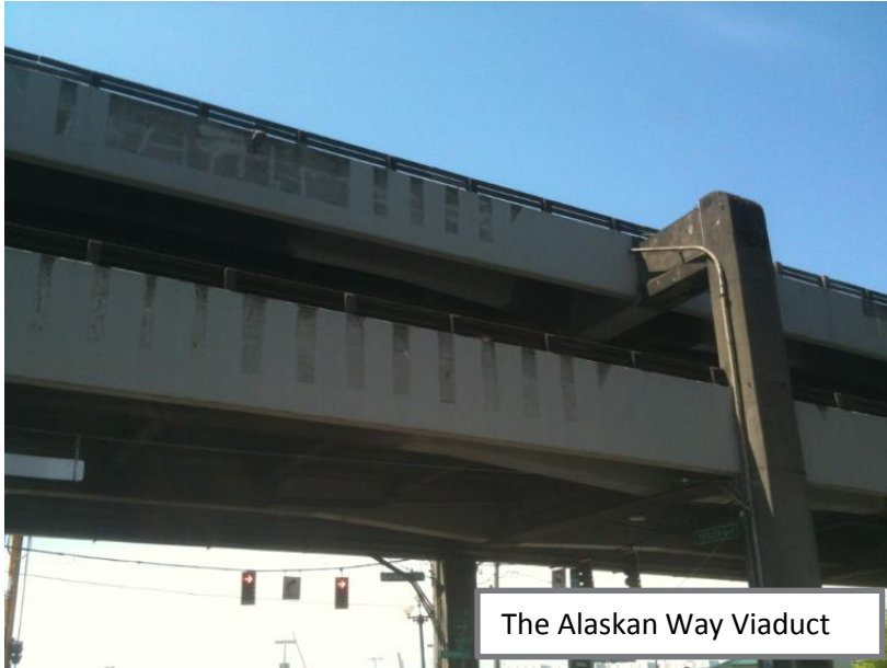
Figure 8: Alaskan Way Viaduct and surrounding areas
