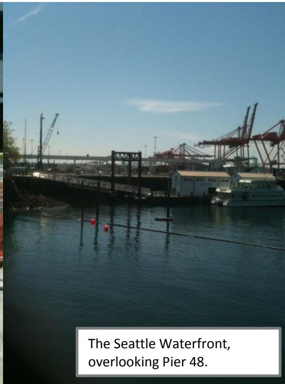
Construction along with Alaskan Way Viaduct
