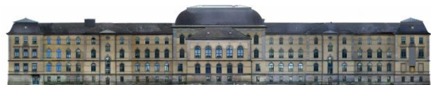
Figure 7. Orthophoto of the town hall's front façade. Image courtesy of Z&M 3D Welt.
