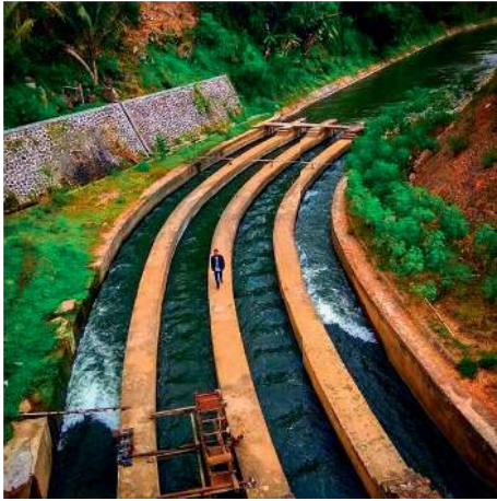
FIGURE 7: Irrigation canal in Bligo village, Ngluwar district, Magelang regency, Central Java province, Indonesia.
