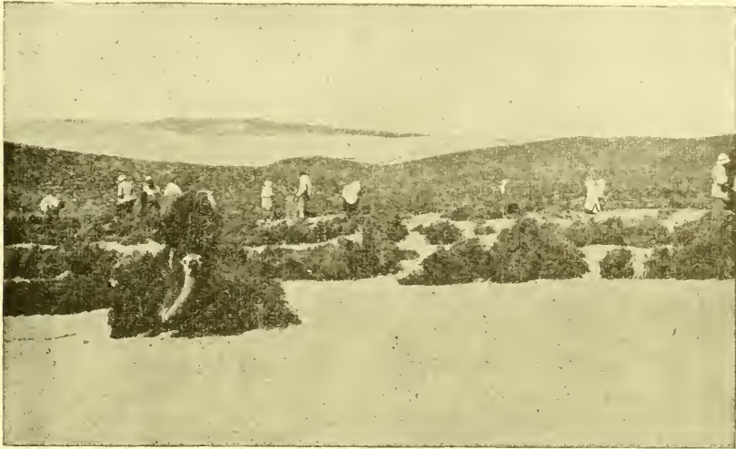
FIG. 163.—Artificial creation of the Ononidetum angustissimae by sowing; first step in fixing sand. (Photo by Maire.)
