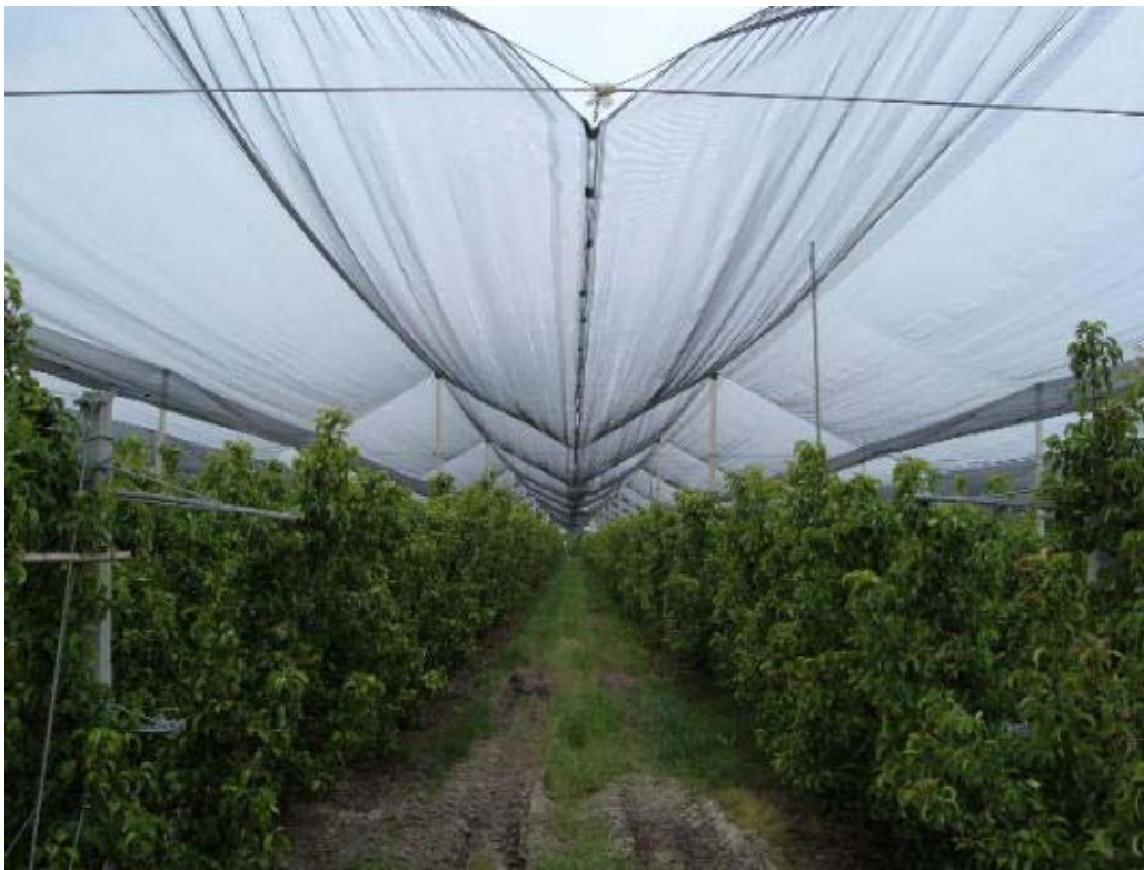
Figure 6. Orchard anti-hail netting on concrete structure in northern Italy.
