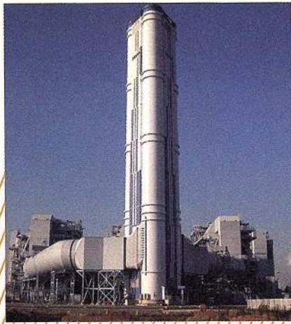
◀ Three Mitsubishi combined cycle plants, far left, generate 1,500 MW at an efficiency of 59 percent and occupy one-third of the land needed by the 40-year-old, 1,050 MW steam plant they replace. One of the new plants is shown in the center photo. The three exhaust through a single stack.
