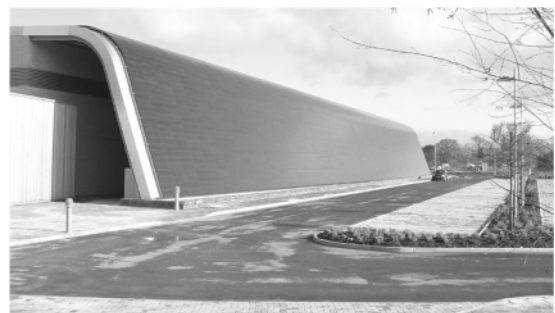
Figure 6: 85-kW thin-film CIS-based BIPV facade, North Wales, UK
