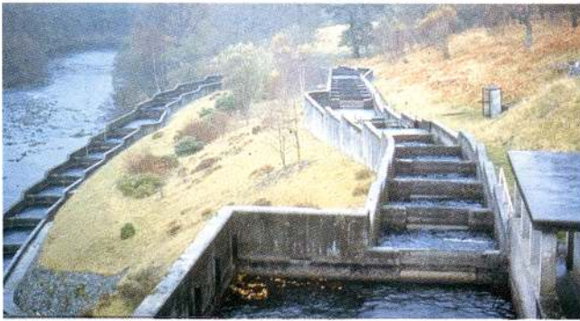
Photo 3: Submerged orifice type fishway at Clunie Dam (Scotland).
