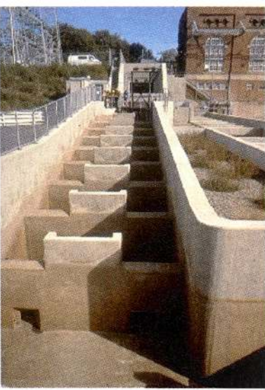
Photo 1: Ice Harbor type fishway at the Vernon dam (Connecticut River, USA), looking upstream.
