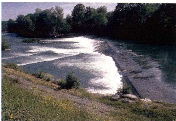
Photo 20 : Pre-barrages at Lestelle weir on the Gave de Pau river
