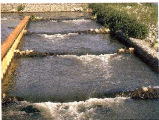
Photo 12: Detail of flow above the V-shaped weir at Sambeck fishway on the river Meuse (Netherlands).
