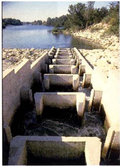
Photo 9: Vertical slot fish pass at a small weir on the river Gardon.
