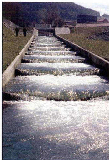
Photo 17: Triangular weir fishway at Sarrancolin dam on the river Neste.
