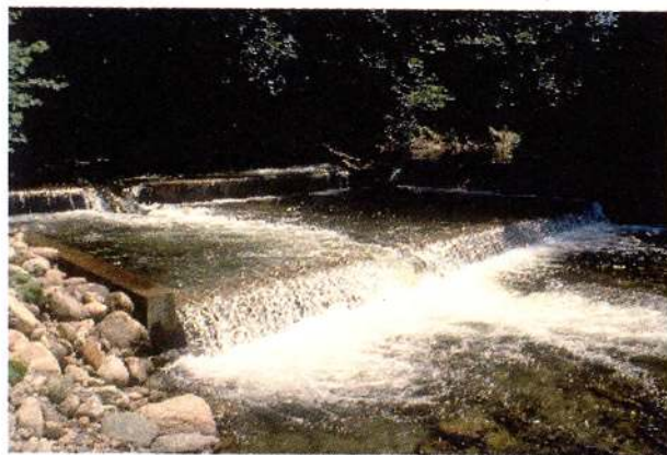
Photo 19: Pre-barrages at Sinsat weir (Ariège river).
