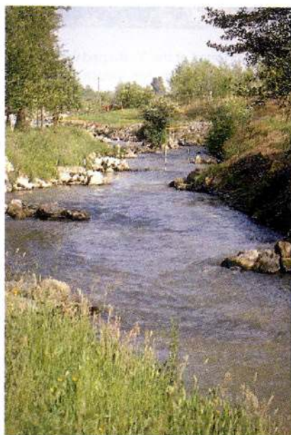
Photo 21: Natural bypass channel at Biron small-scale power plant on the Gave de Pau river.
