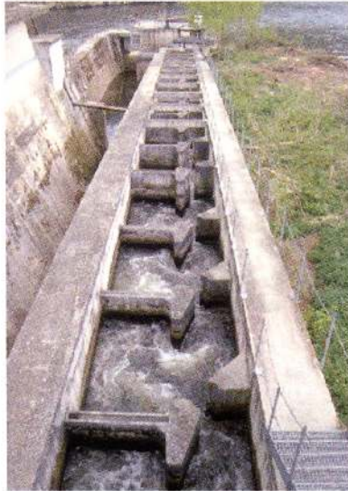
Photo 8: Vertical slot fishway at Mauzac power plant on the river Dordogne.
