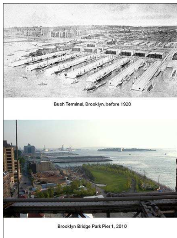
Figure 7.15 Photographs of the former and current uses of the Brooklyn Bridge Park site, Brooklyn. One of the piers shown in the top picture was demolished and converted into a public park.
