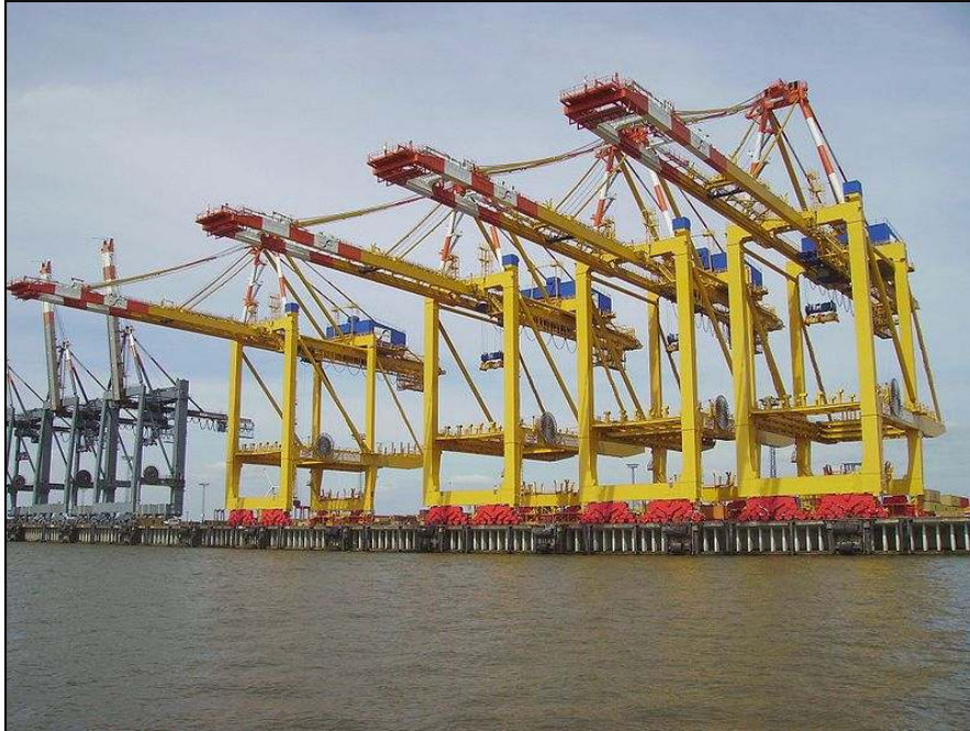
Figure 6.4 Container cranes at the container-terminal of Bremerhaven in Germany. 2009. Photograph. Cargo ships dock under these cranes. The cranes remove metal box containers from the ships and transport them to waiting trucks or rail cars.
