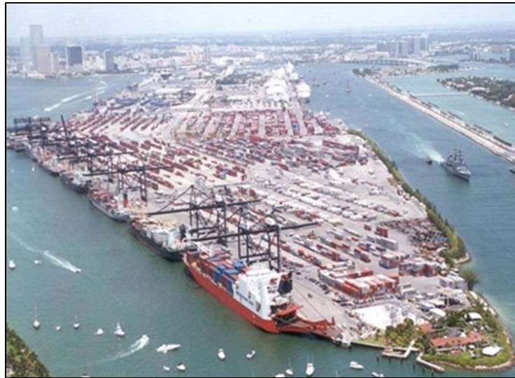
Figure 2.3 Port of Miami, Florida. 1995. Photograph. This photograph shows a modern and extensive port facility constructed away from the city's downtown. Specialty cranes remove cargo containers from ships to awaiting vehicles for transport.
