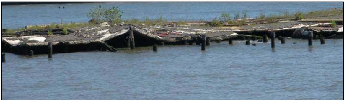
Figure 6.7 Rotted pier in the Hudson River, Hoboken. 2011. Personal photograph by author. This pier was once used for the transference of cargo from ships on the Hudson River to the shores of Hoboken, New Jersey.
