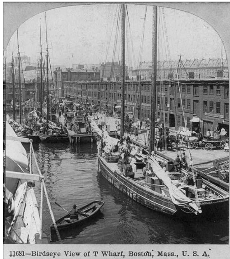
Figure 2.2 Bird's-eye view of T Wharf, Boston, Mass. 1910. Photograph. B.L. Singley (Keystone View Co.). The photograph illustrates how boats loaded with cargo moored along long wharves and unloaded onto waiting horse drawn carts.
