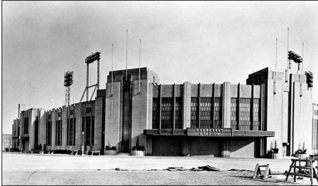
Figure 10.9 Roosevelt Stadium, New Jersey. Main entrance from west, ca. 1940. Photograph. The stadium sat on the Newark Bay waterfront in Jersey City.
