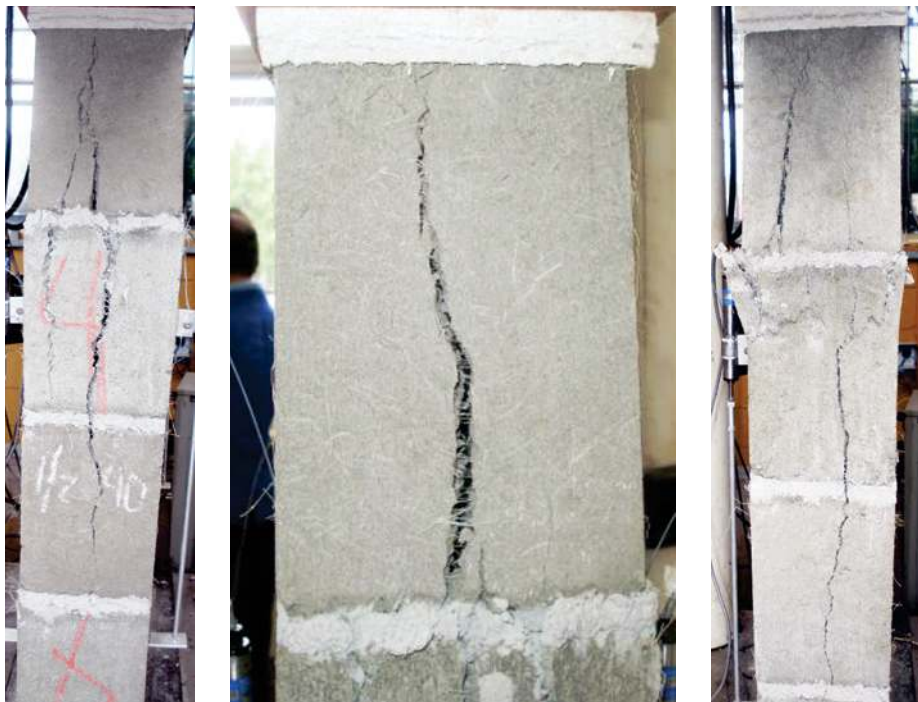
Figure 16 – Vertical cracks developed along the lateral septa
