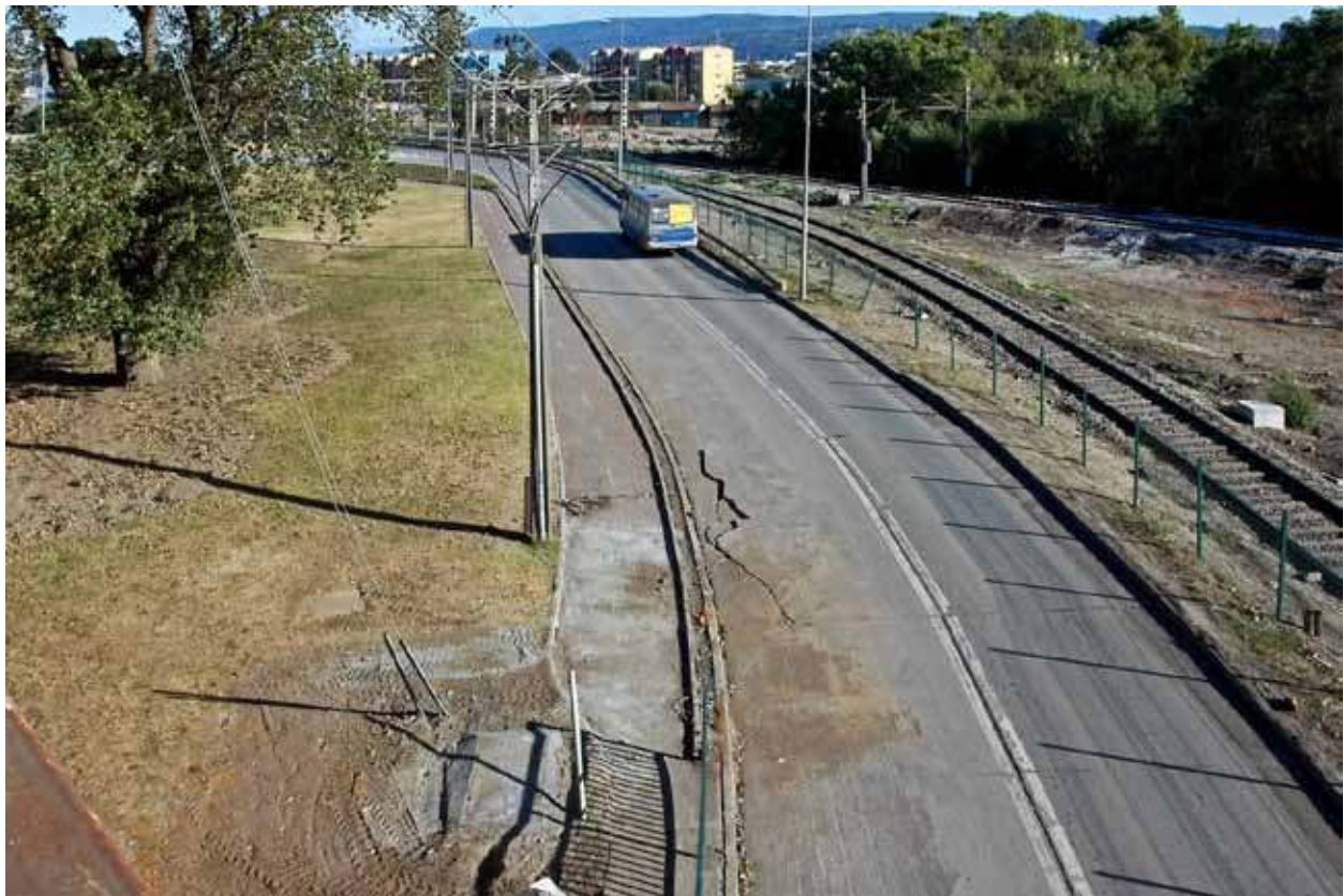
Figure 273. Photo. Possible liquefaction features near wall site 28C.
