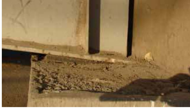
Figure 161. Photo. Steel girder on neoprene pad at abutment of Route 5 pedestrian bridge.
