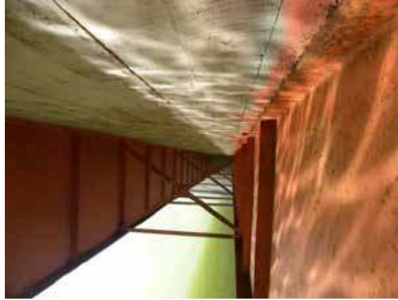
Figure 142. Photo. Web stiffeners in Pichibudis bridge.
