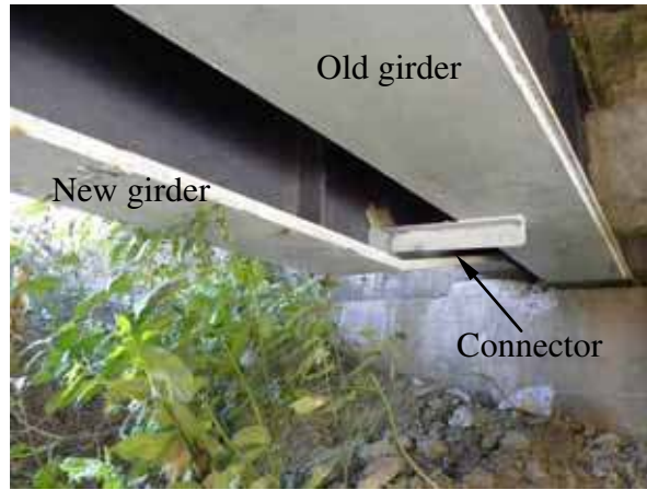
Figure 150. Photo. Retrofit girder connections on El Bar bridge.
