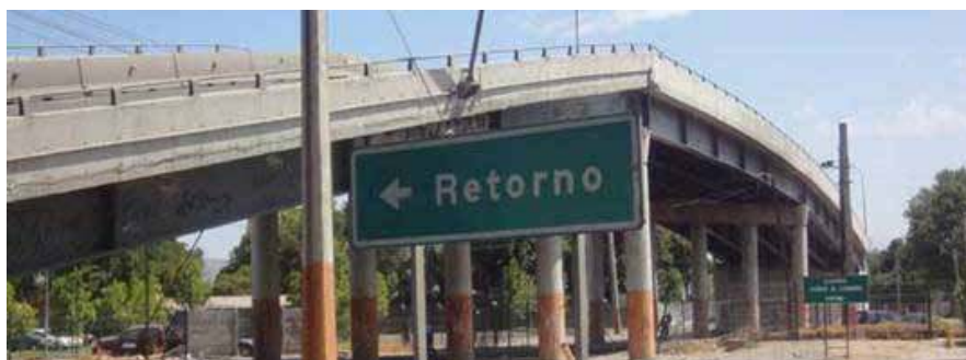
Figure 106. Photo. Overview of Quilicura railway overcrossing.
