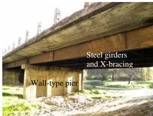
Figure 77. Photo. Overview of west Ramadillas bridge.
