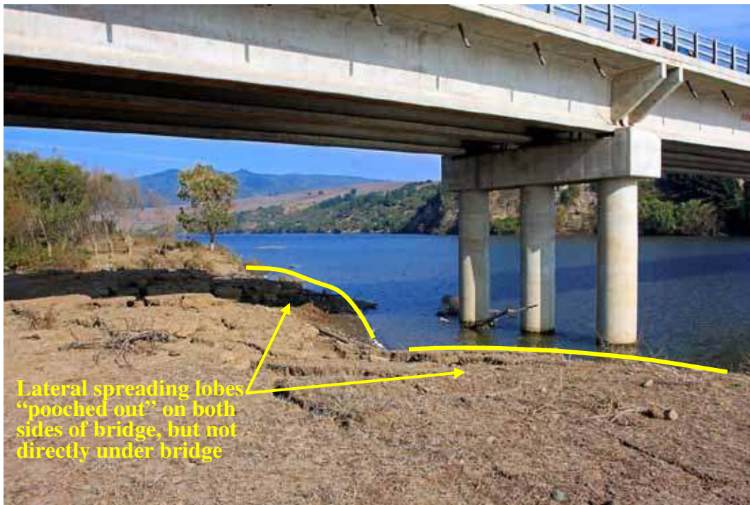
Figure 193. Photo. Lateral spreading at Mataquito bridge with lateral movement beneath and around bridge.
