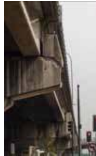
Figure 31. Photo. Westbound Independencia bridge.
