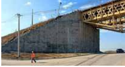
Figure 252. Photo. Retaining wall at Maipú River bridge.
