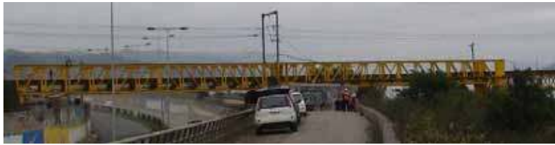
Figure 171. Photo. North end of Chepe railroad bridge over roadway.
