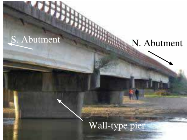
Figure 73. Photo. Side view of east Ramadillas bridge.
