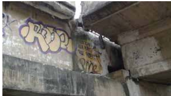
Figure 50. Photo. Interior face of westbound ramp to Llacolen bridge at the river end.
