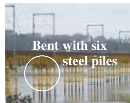
Figure 172. Photo. River spans of Chepe railroad bridge.
