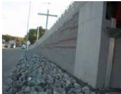
Figure 259. Photo. Retaining wall at Rotonda General Bonilla.
