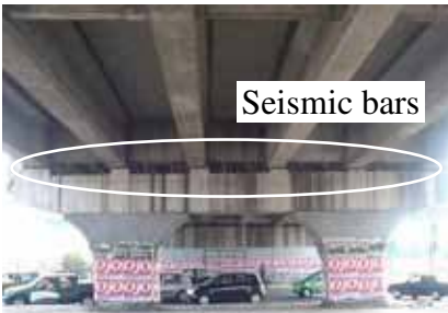
Figure 27. Photo. Typical flared wall pier of westbound Independencia bridge.
