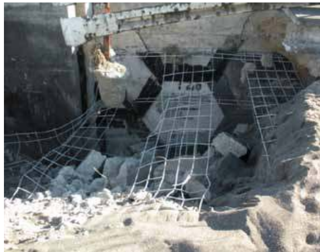
Figure 270. Photo. Back side of upper wall at wall site 28C.
