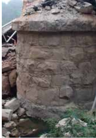
Figure 169. Photo. Foundation of Claro River bridge.
