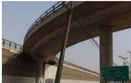
Figure 32. Photo. Entrance ramp to westbound Independencia bridge.
