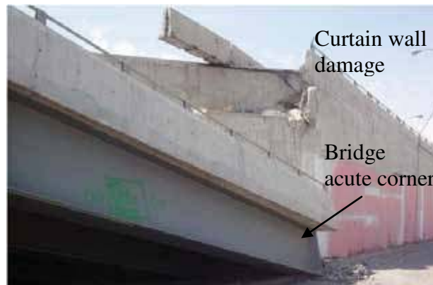
Figure 109. Photo. East abutment of Quilicura railway overcrossing.
