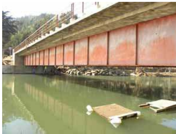
Figure 141. Photo. Cross frames in Pichibudis bridge.
