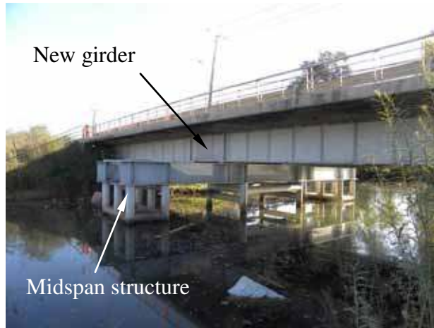
Figure 149. Photo. Side view of El Bar bridge.
