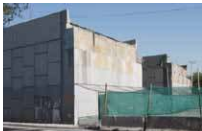
Figure 246. Photo. Retaining wall at Américo Vespucio/Miraflores.
