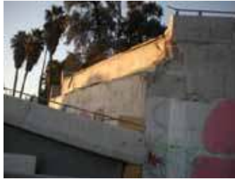
Figure 249. Photo. Retaining wall at Quilicura railroad overcrossing.
