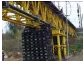
Figure 173. Photo. South end of Chepe railroad bridge.
