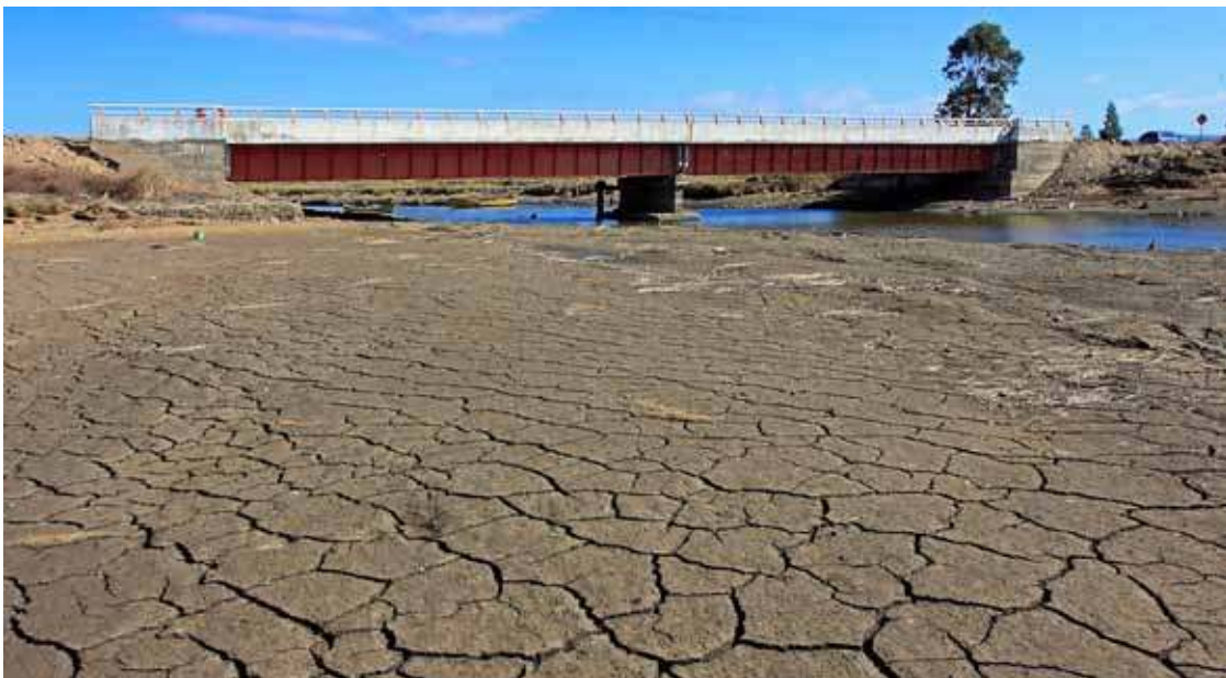
Figure 207. Photo. Raqui 1 bridge viewed from north side.
