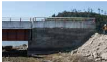
Figure 255. Photo. Retaining wall at Raqui 2.
