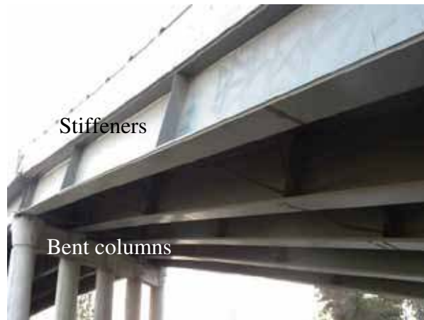
Figure 108. Photo. Stiffeners on Quilicura railway overcrossing.
