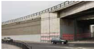
Figure 250. Photo. Retaining wall at Américo Vespucio/Independencia eastbound.
