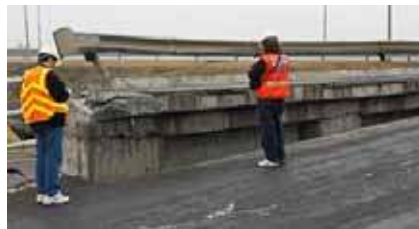
Figure 256. Photo. South retaining wall at Juan Pablo II.
