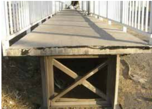
Figure 162. Photo. End cross frame near collapsed span of Route 5 pedestrian bridge.
