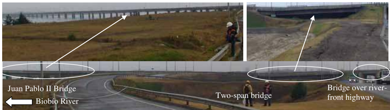
Figure 59. Photo. Approaches to Juan Pablo II bridge.
