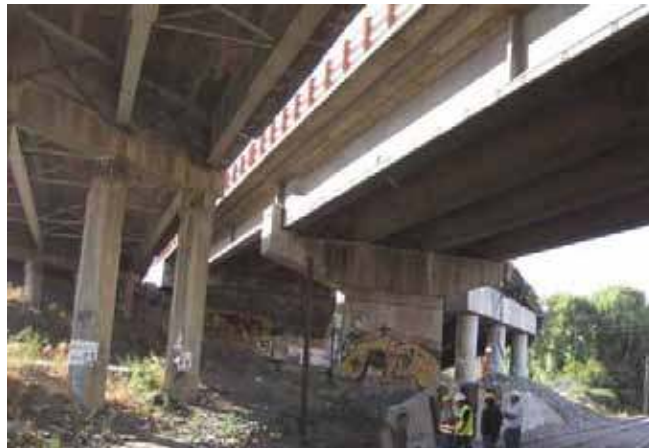
Figure 102. Photo. Three bridges (one demolished) at Route 5 overcrossing at Hospital.
