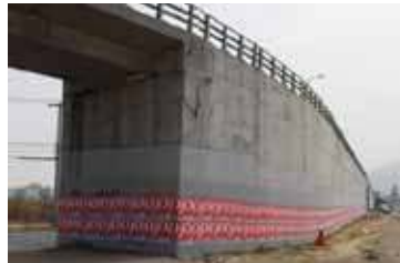
Figure 251. Photo. Retaining wall at Américo Vespucio/Independencia westbound.
