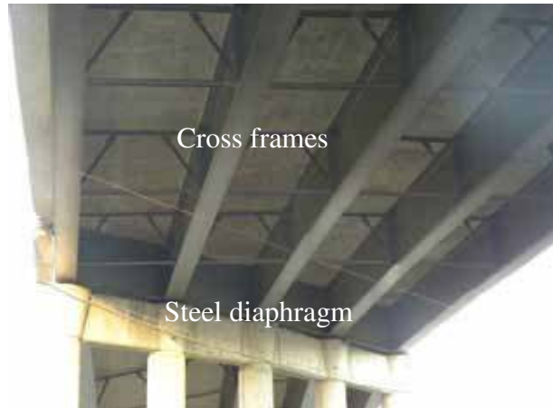
Figure 107. Photo. Cross frames on Quilicura railway overcrossing.
