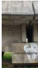
Figure 51. Photo. Bent of westbound ramp to Llacolen bridge.
