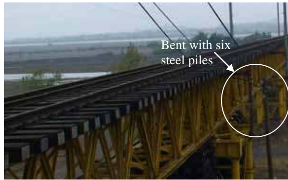
Figure 175. Photo. Section on south end of Chepe railroad bridge.
