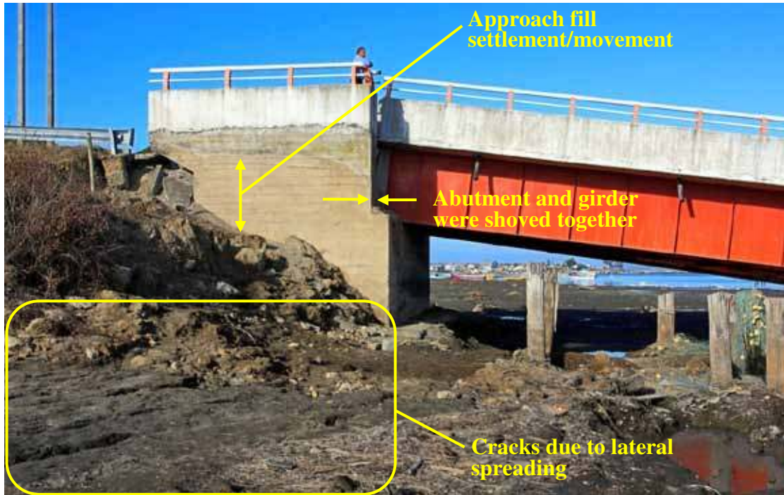
Figure 240. Photo. Overview of Tubul bridge north abutment.
