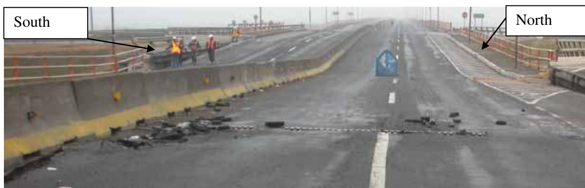
Figure 265. Photo. Wall settlement near Juan Pablo II bridge due to liquefaction-induced settlement.
