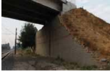
Figure 253. Photo. Retaining wall at Estribo Francisco Mostazal (Avenida Independencia).
