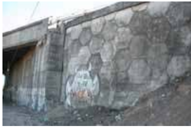
Figure 258. Photo. Retaining wall at 21 de Mayo.
