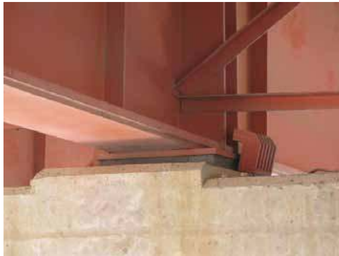
Figure 124. Photo. Elastomeric pad and stopper over bent on Cardenal Raúl Silva Henríquez bridge.
