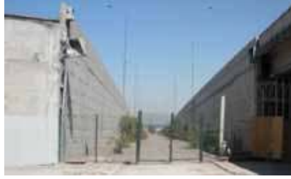
Figure 247. Photo. Retaining wall at Américo Vespucio/Lo Echevers.
