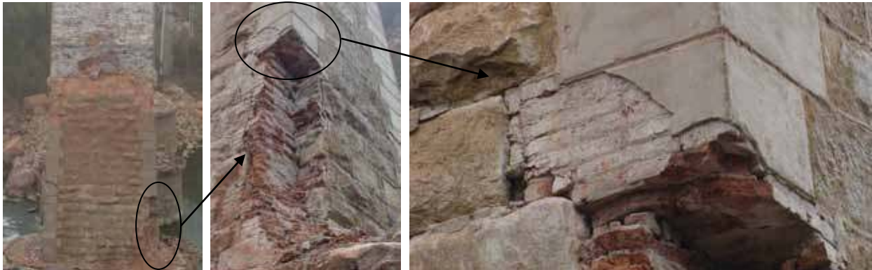
Figure 168. Photo. Pier of Claro River bridge.
