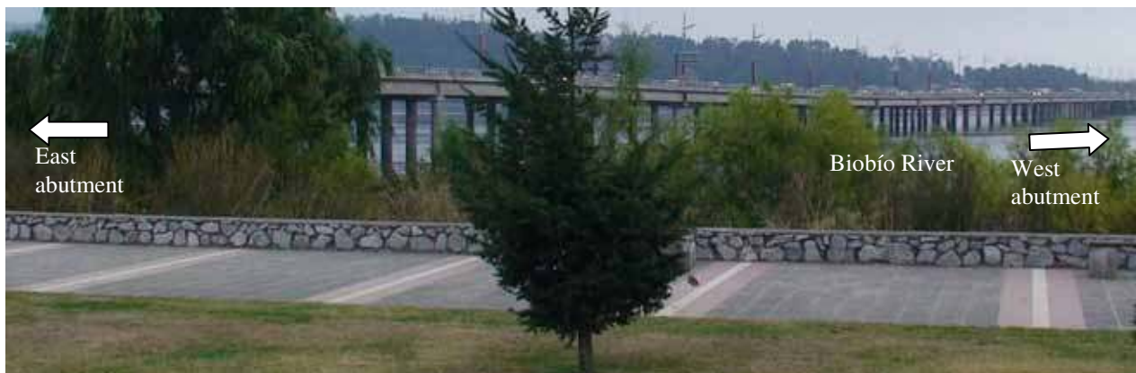
Figure 42. Photo. Llacolen bridge looking south-southwest.
