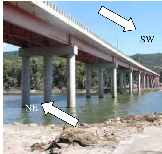
Figure 123. Photo. Cardenal Raúl Silva Henríquez bridge looking south.
