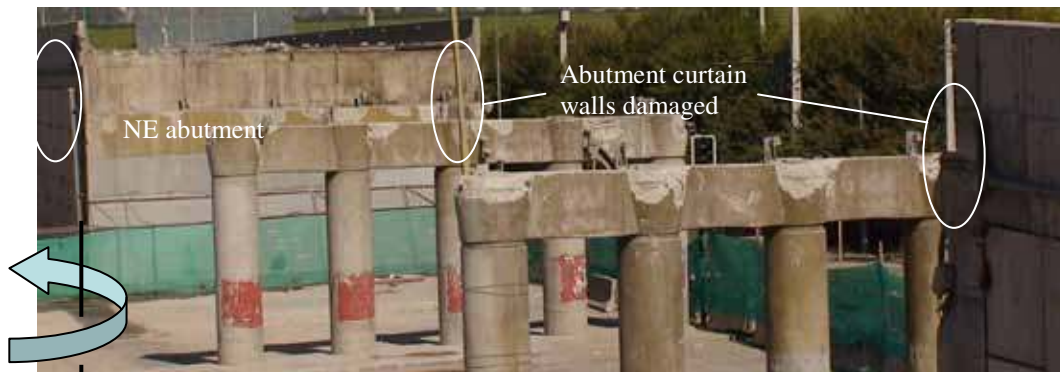
Figure 89. Photo. Miraflores bridge after removal of superstructure.
