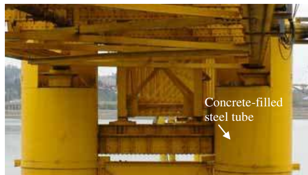
Figure 174. Photo. Bottom view and cross section on north end of Chepe railroad bridge.
