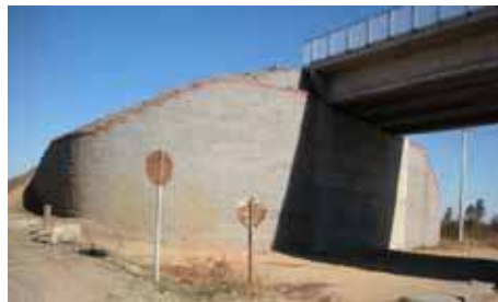
Figure 260. Photo. Retaining wall at Muros Talca (SW).
