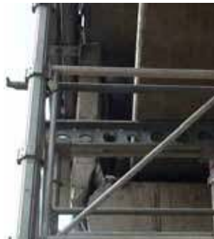
Figure 24. Photo. Curtain wall at east abutment of eastbound Independencia bridge.
