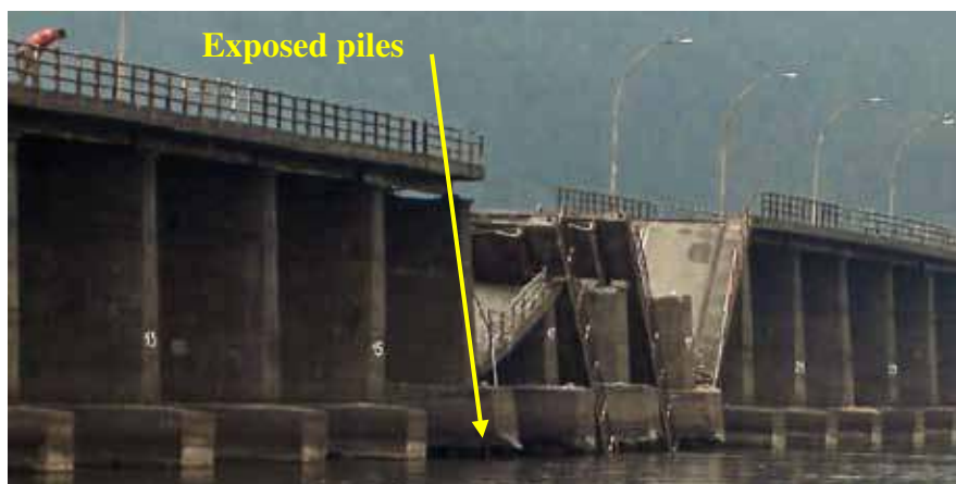
Figure 224. Photo. Close-up of old Biobío River bridge showing exposed pile foundations.
