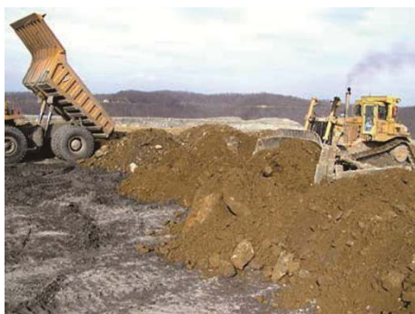
(a) Placement of brown topsoil up to 1.5 m in depth
