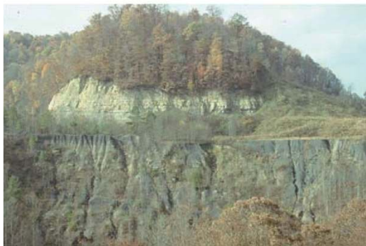
(c) An acidic outcrop and highwall left by a pre-law contour mining in Virginia
