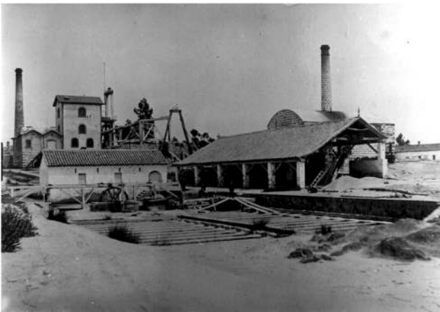
Fig. 12 Mining and ore dressing installations of Palmerston shaft at the end of nineteenth century
