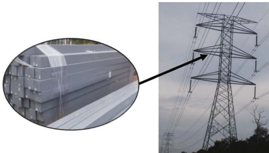
FIGURE 10: Potential application of green composite in cross arm beams.
