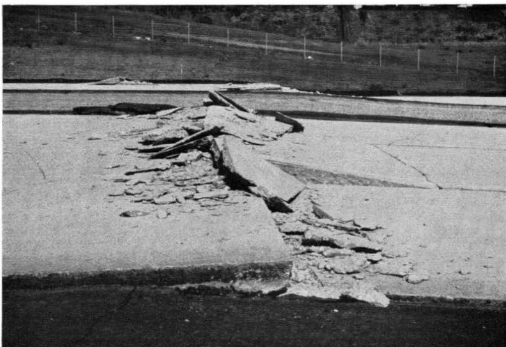
Fig. 24. 1971 San Fernando, California thrust fault break passing through concrete pavement showing buckling resulting from shortening of a distance between points on opposite sides
