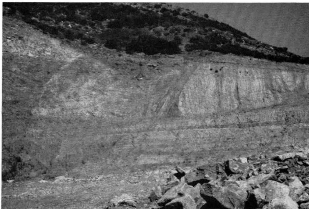
Fig. 17. Cedar Springs Dam during construction showing fault No. 1 exposed in excavation in east abutment at location shown in Fig. 12
