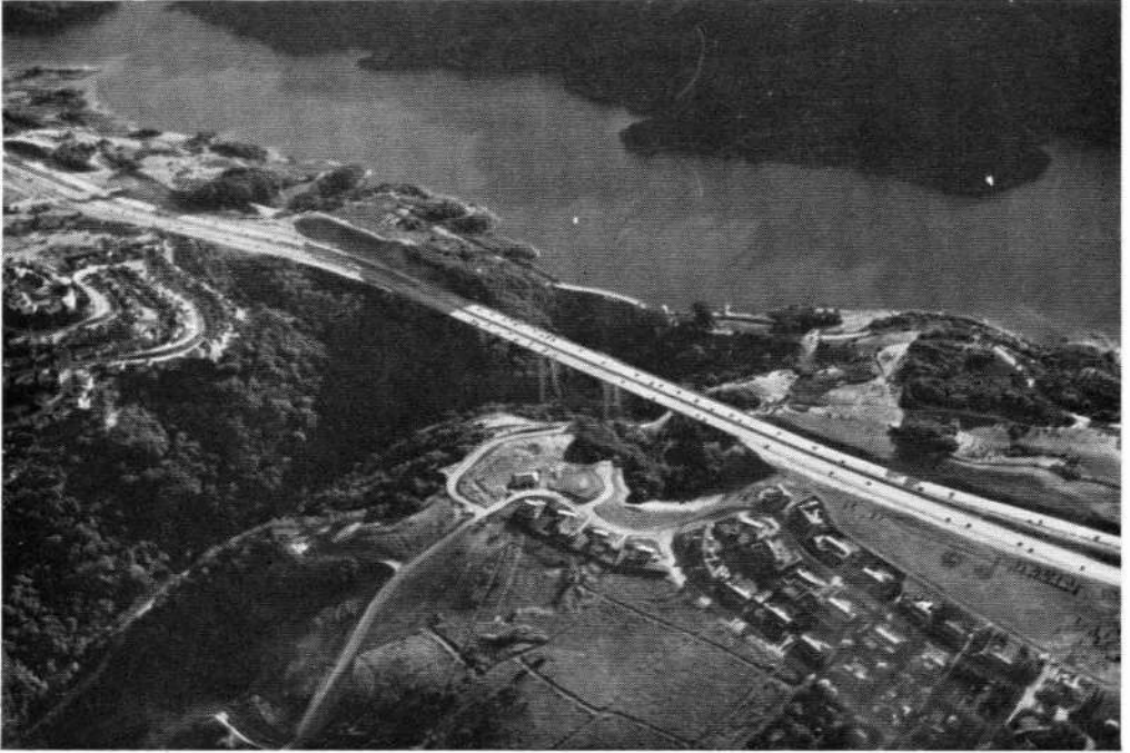
Fig. 3. Looking west at the Lower Crystal Springs Dam. The 43 m high concrete gravity dam retains a 65 million m 3 water supply reservoir in the north-south rift valley of the San Andreas Fault. The dam closes a gorge in the east wall of the valley and is off the fault. The 1906 break on the fault passed near the centre of the reservoir, running parallel with the longitudinal axis of the dam about 200 m upstream
