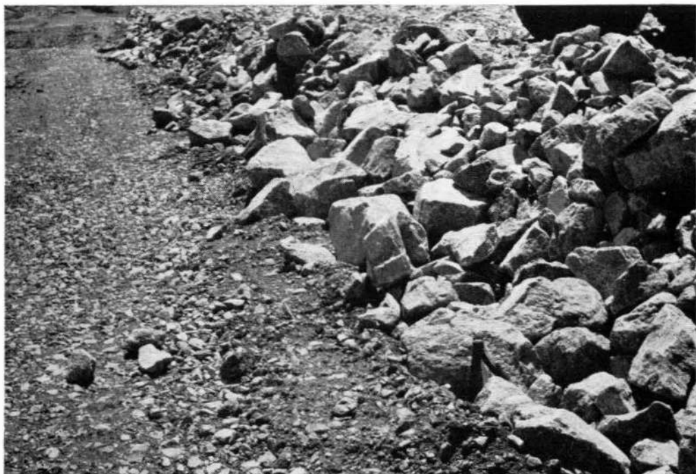
Fig. 16. Cedar Springs Dam during construction, looking at the boundary between transition zone 3 and downstream rockfill zone 4. It is apparent that the permeability of rockfill zone 4 is several orders greater than that of zone 3
