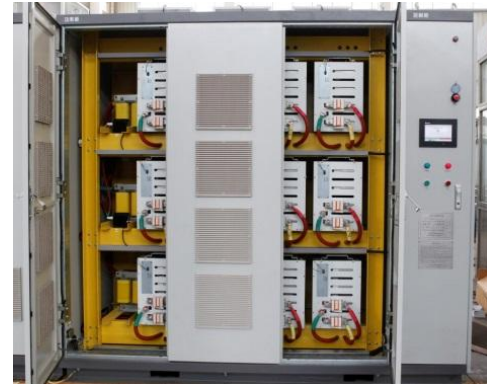
(b) Nine-level high voltage inverter
