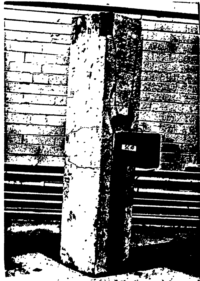
Figure 3.14 Specimen SC10 - 1 1/2 in (38 mm) concrete cover; the load deflection response and a photograph of the specimen after failure
