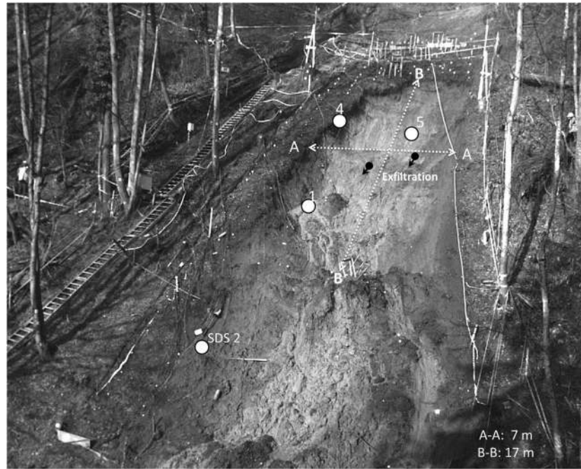
Fig. 7 Post event record of the landslide and relative location of the soil deformation sensors with respect to the destabilised soil mass
