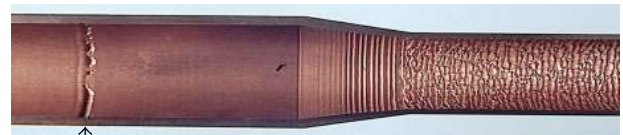
Lap joint close to seal weld
