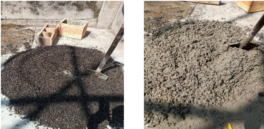
Fig. 4 Mixing of Palm Kernel Shell Concrete
